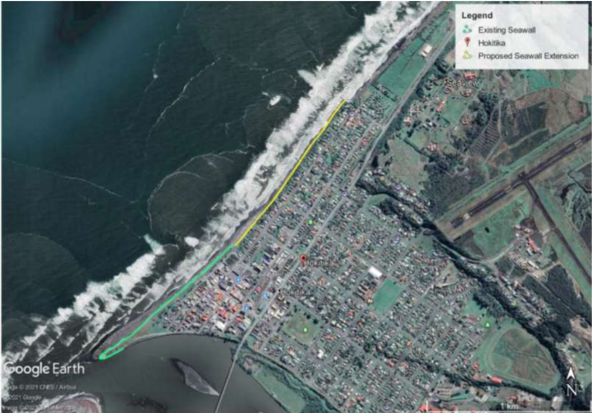
Figure 1 Location of existing Hokitika seawall and proposed seawall extension
