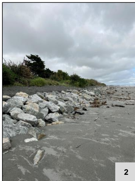
Photo 2: Temporary seawall in the form of large boulders (facing south-west). Sand deposits can be seen washed up behind the boulders.
