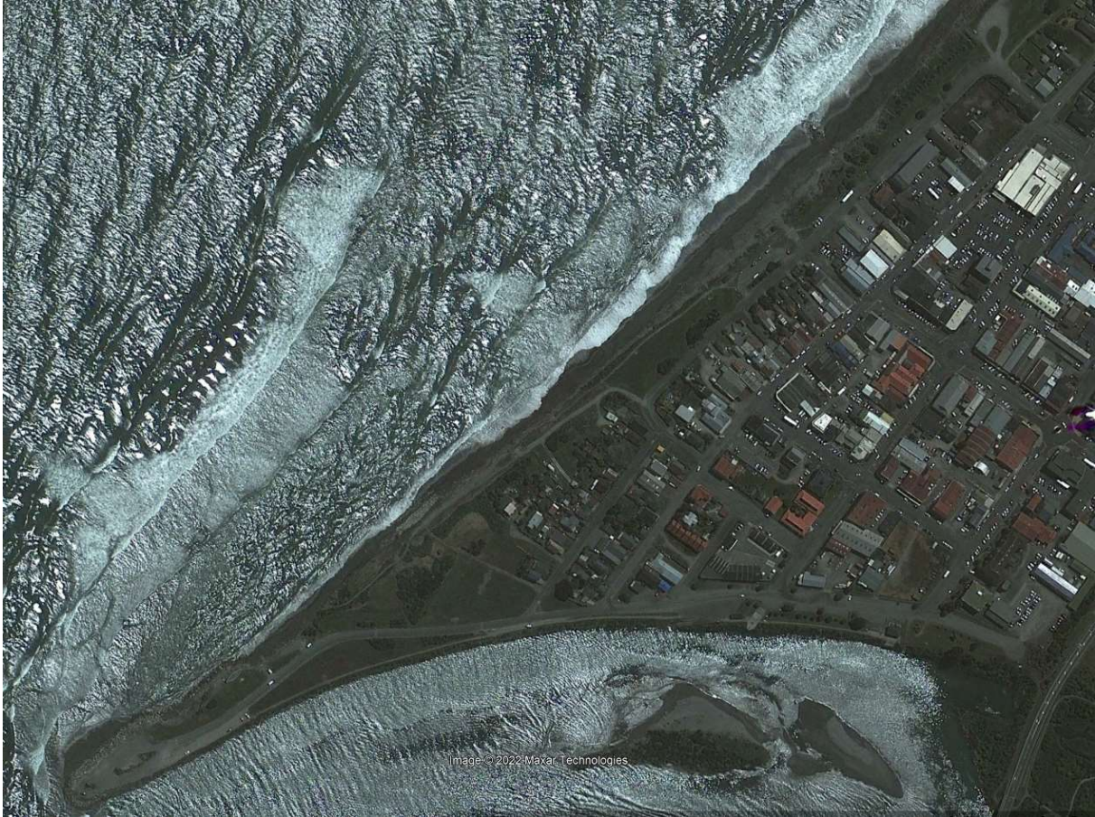
Figure 1a: Existing revetment, December 2012 (from GoogleEarth)
