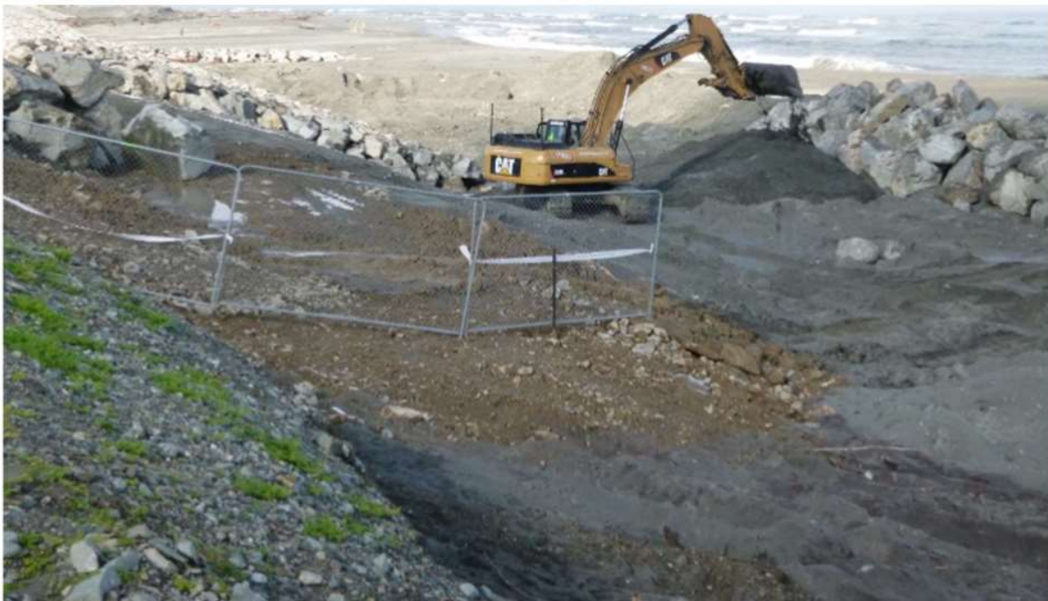
Figure 3-4 Installation of existing seawall showing temporary sand bund and rock stockpile
