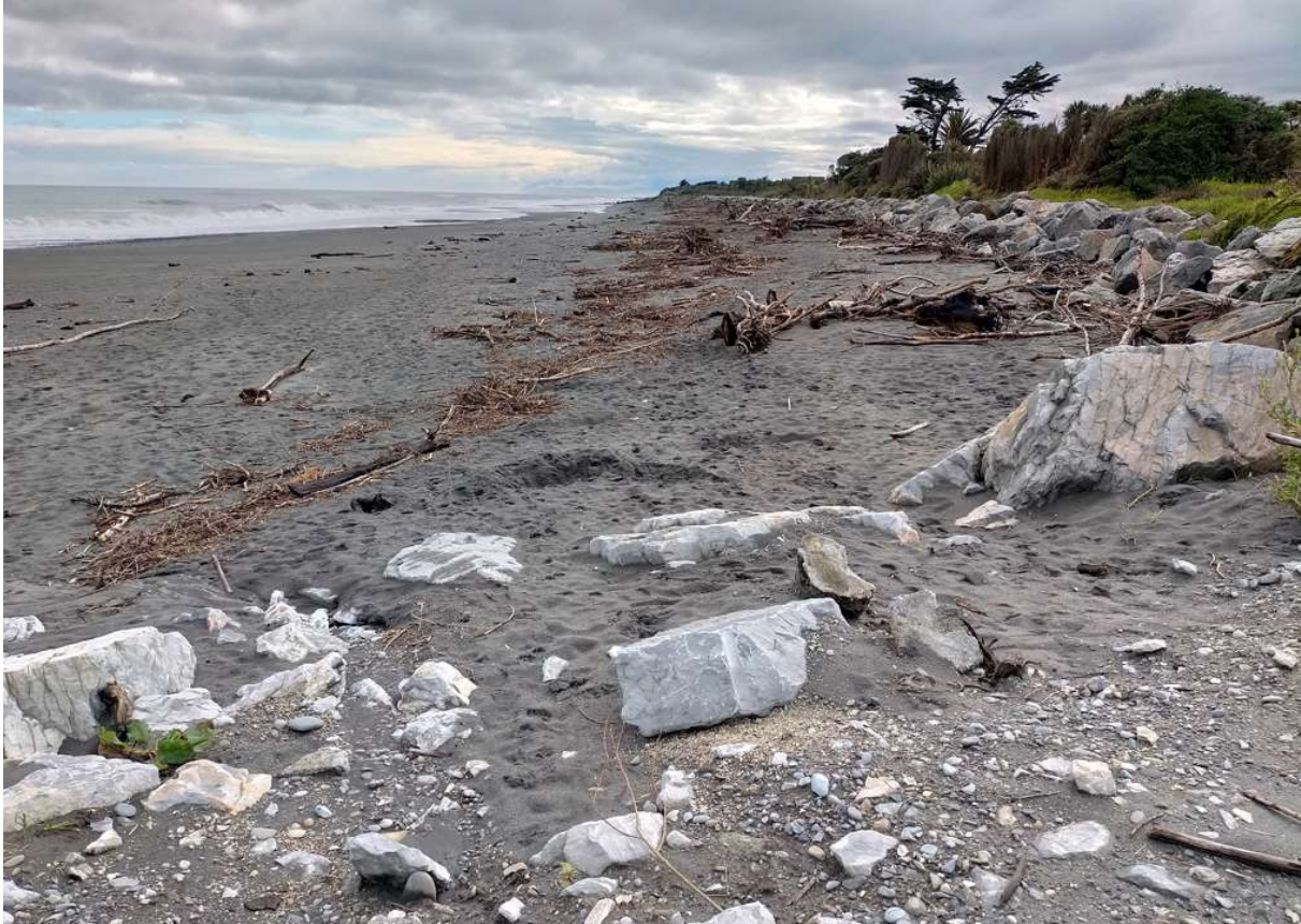
Figure 3-1 Wave runup (illustrated by driftwood) to existing seawall
