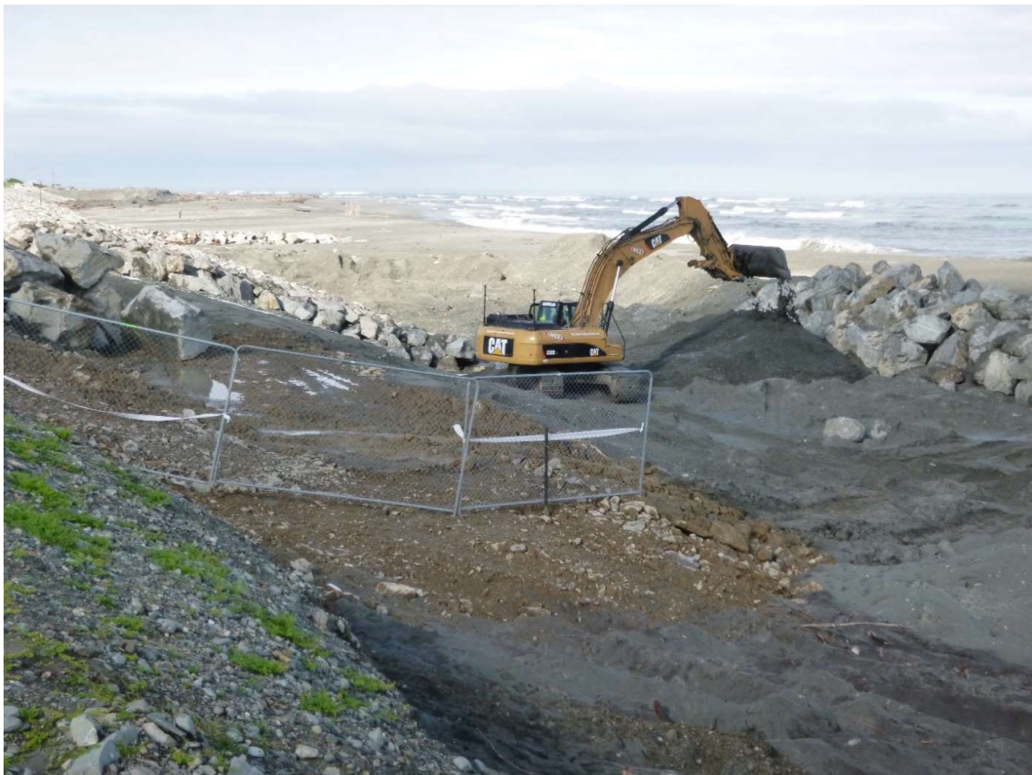
Figure 3-4 Installation of existing seawall showing temporary sand bund and rock stockpile
