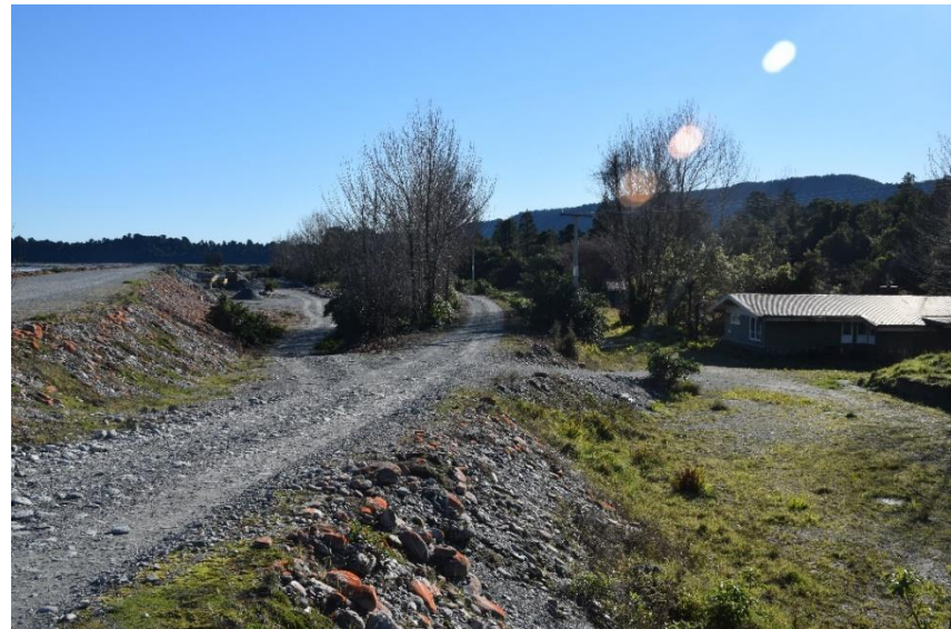
Figure 1-5 - Old bank adjacent to new Havill Wall Bank
