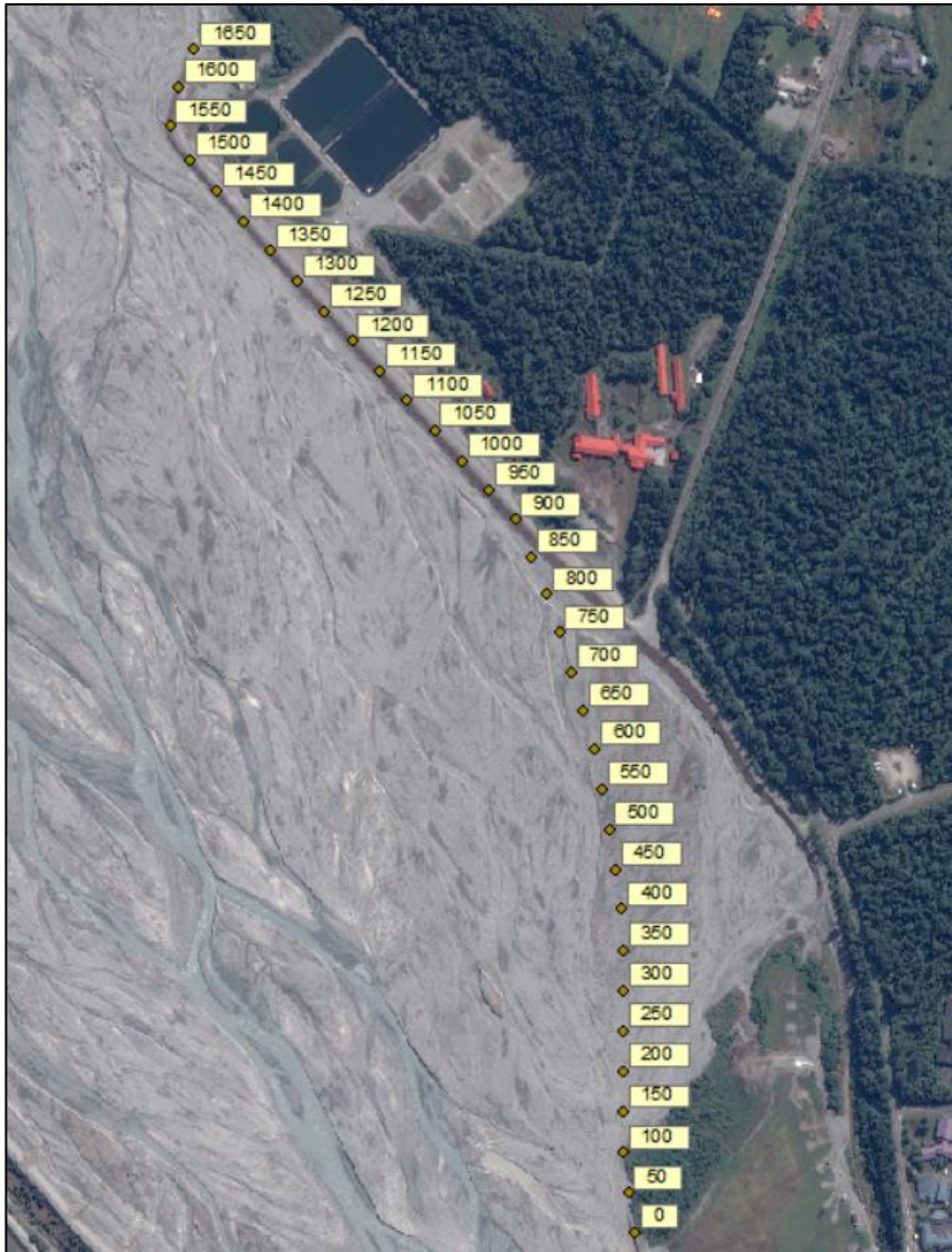
Figure 0-4 - Bank 2 - Alignment B distance marker
