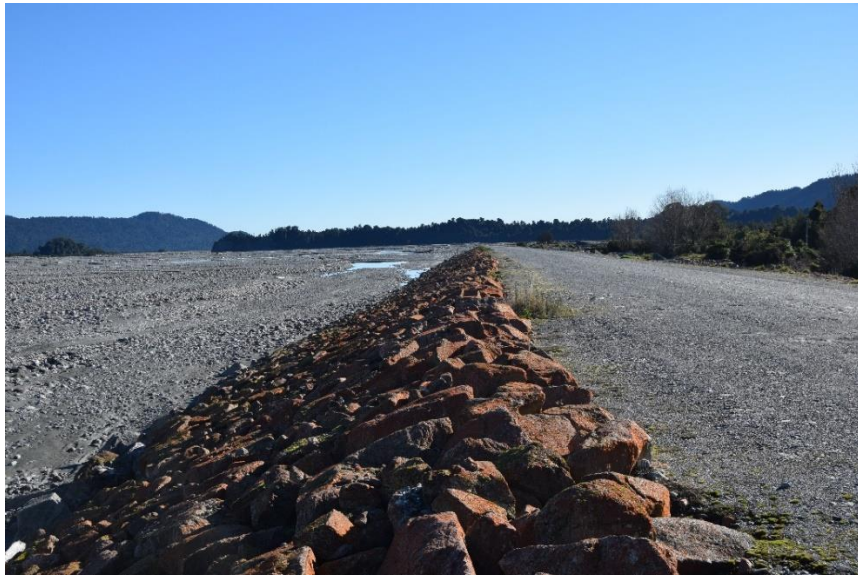
Figure 1-2 - View downstream of the existing rock on the Havill Wall Bank.
