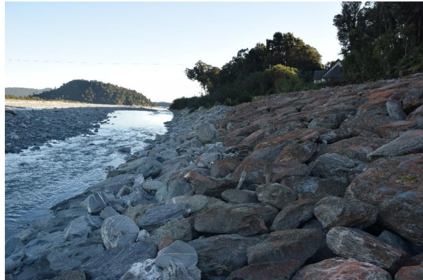
Figure 1-3 - Rock lining on the Church bank
