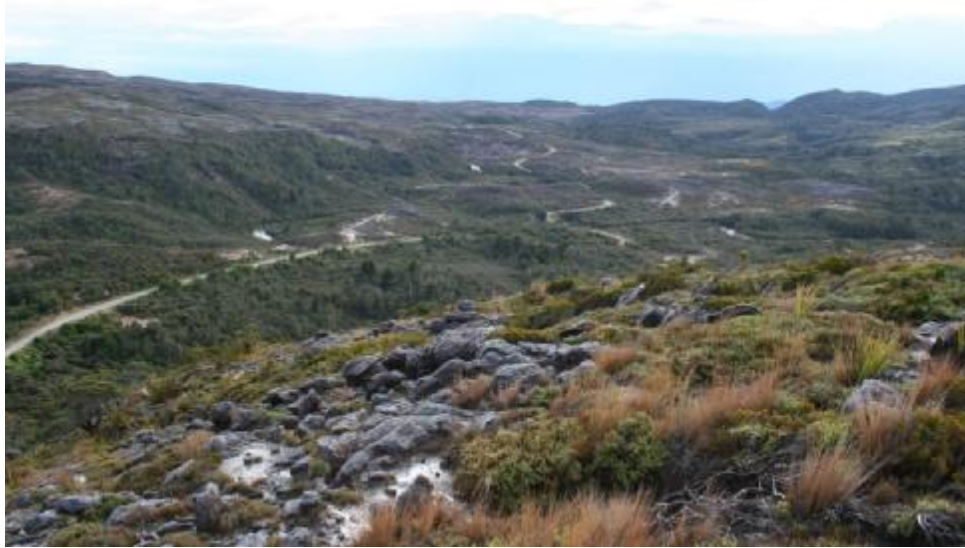
Figure 2: Looking over the proposed Lake William retention pond area in the foreground and down the path of the proposed pipeline towards the Mangatini Stream.
