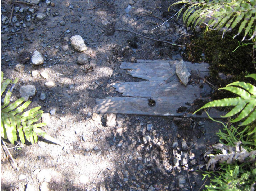
Plate 2: Remains of sleeper on formation of Electric Locomotive Line, Stockton Plateau. Weka Creek section, 3 March 2009 (Janine Dunlop, NZHPT, Southern Regional Office)
