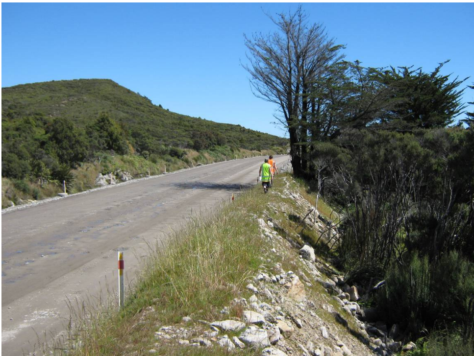
Plate 3: Section of Haul Road at site of Tintown settlement. Cutting for Electric Locomotive Line situated on the left side of the road embankment; Tintown situated at right (remains of fireplace located at stand of exotic trees at the centre-right of the image), 3 March 2009 (Janine Dunlop, NZHPT, Southern Regional Office)
