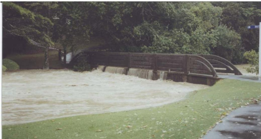
Sawyers Creek floodwaters lapping the footbridge in Dixon Park, Greymouth on January 24<sup>th</sup> 2000. Before major floodworks were completed upstream in the 1970’s this creek had been known to top this bridge. *Both photographs by M Shearer, WCRC Engineer*
