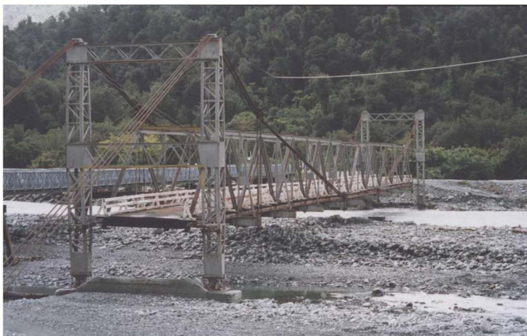
Note how low the suspension bridge, since removed, is to the water. Bailey bridge in background
