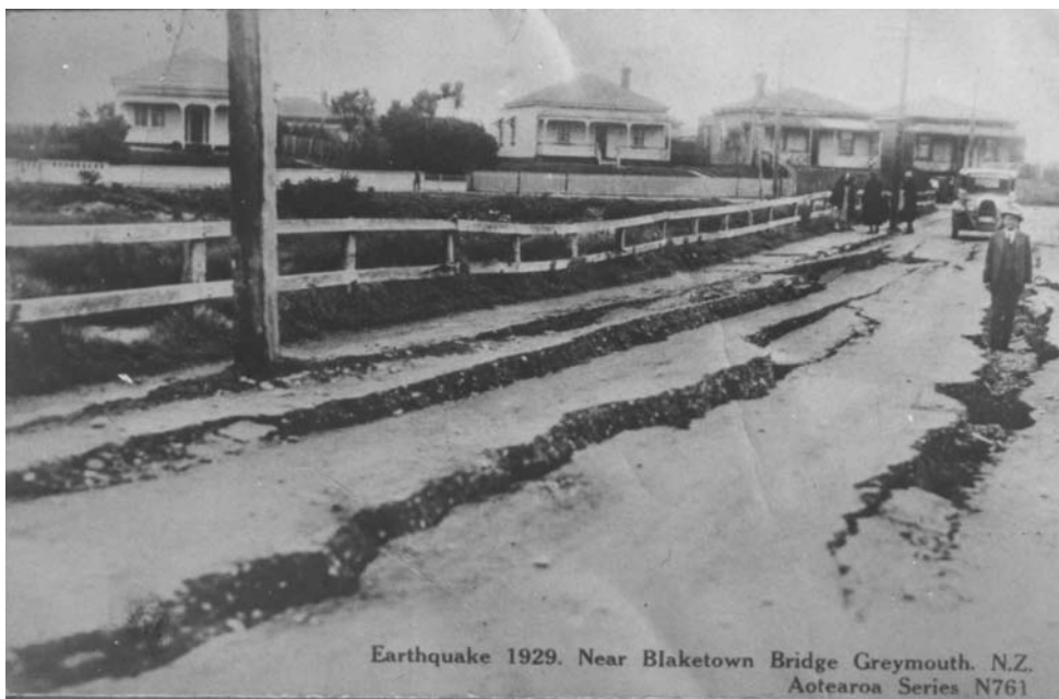
This picture was taken in Preston Road. The road fissures have been caused by liquefaction of the sandy soils in the Blaketown area.
