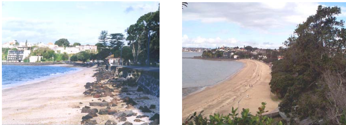
Figure 1. Mission Bay Auckland with seawall and rock armour (negative environmental outcome) and after it was renourished with sand from Pakiri Beach (positive environmental outcome).
