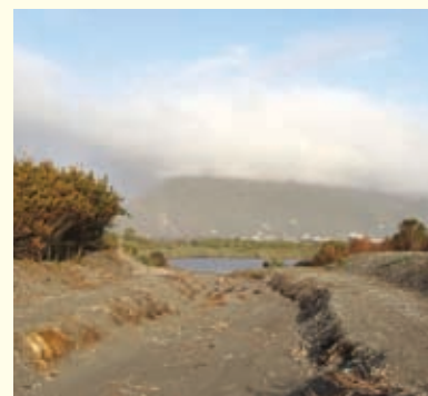
A view of the newly widened Cobden 'cut' taken from the beach and looking back toward the lagoon. If necessary, the beach can be excavated to allow for floodwaters to drain away.
