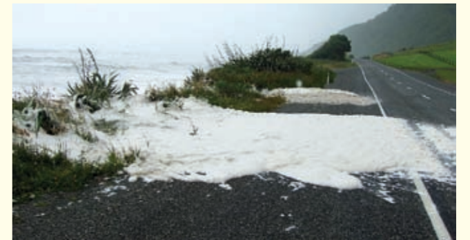
High seas associated with spring tides and stormy weather spilled over onto the Coast Road north of Greymouth in January 2006.
