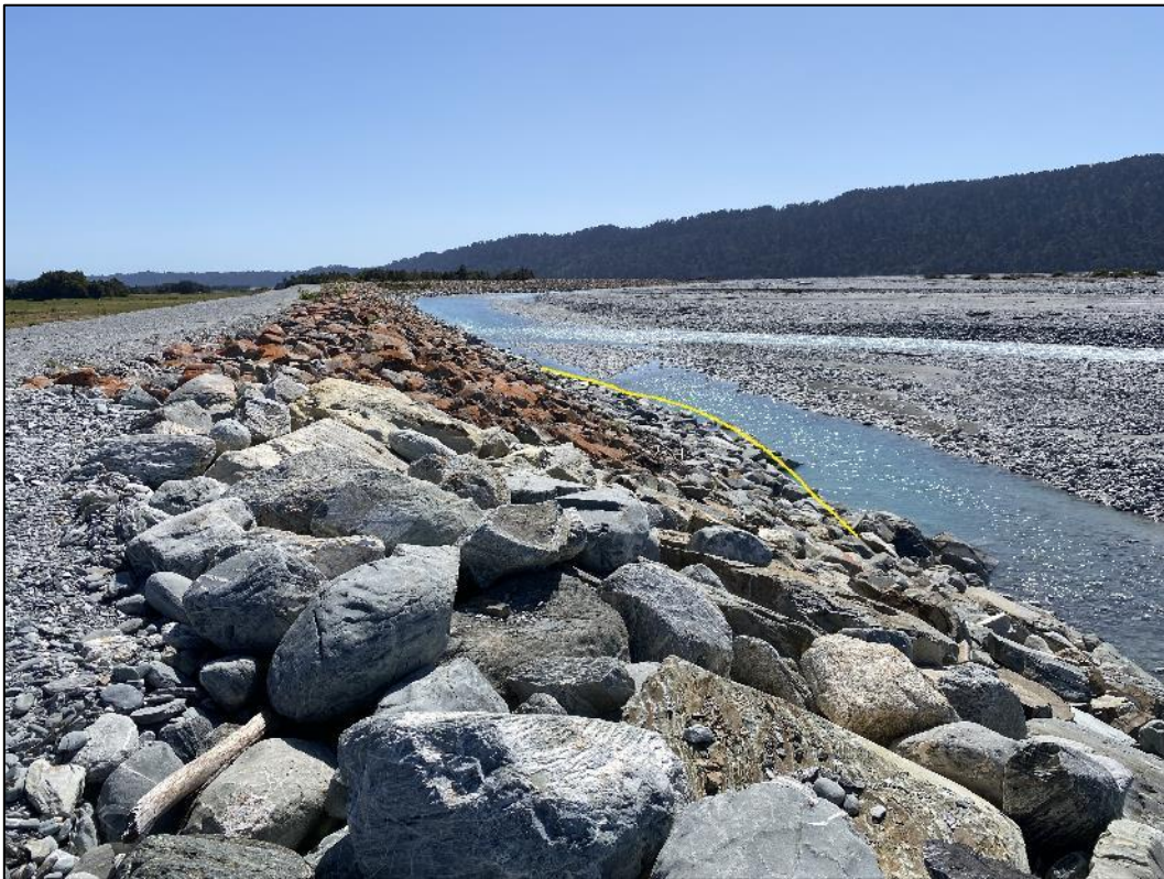
Figure 4-8 - Visible stopbank slumping (highlighted in yellow)
