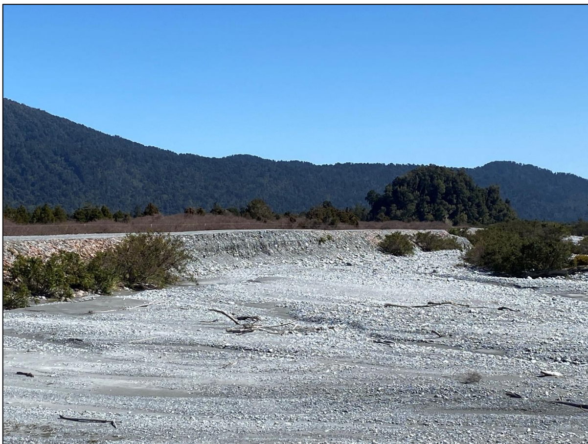
Figure 4-7 – Example of erosion on true left bank (photo taken in October 2022)
