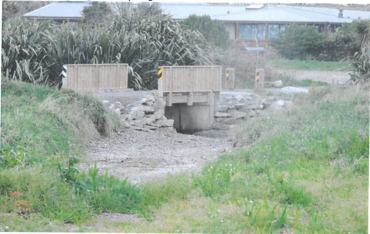
Photo 2: Bridge after outlet opened.
