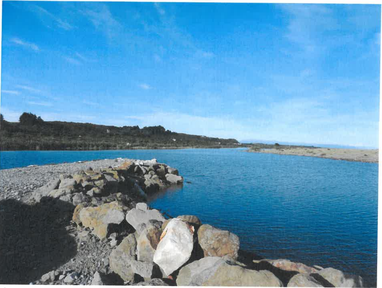
Photo 3: New River before opening.
