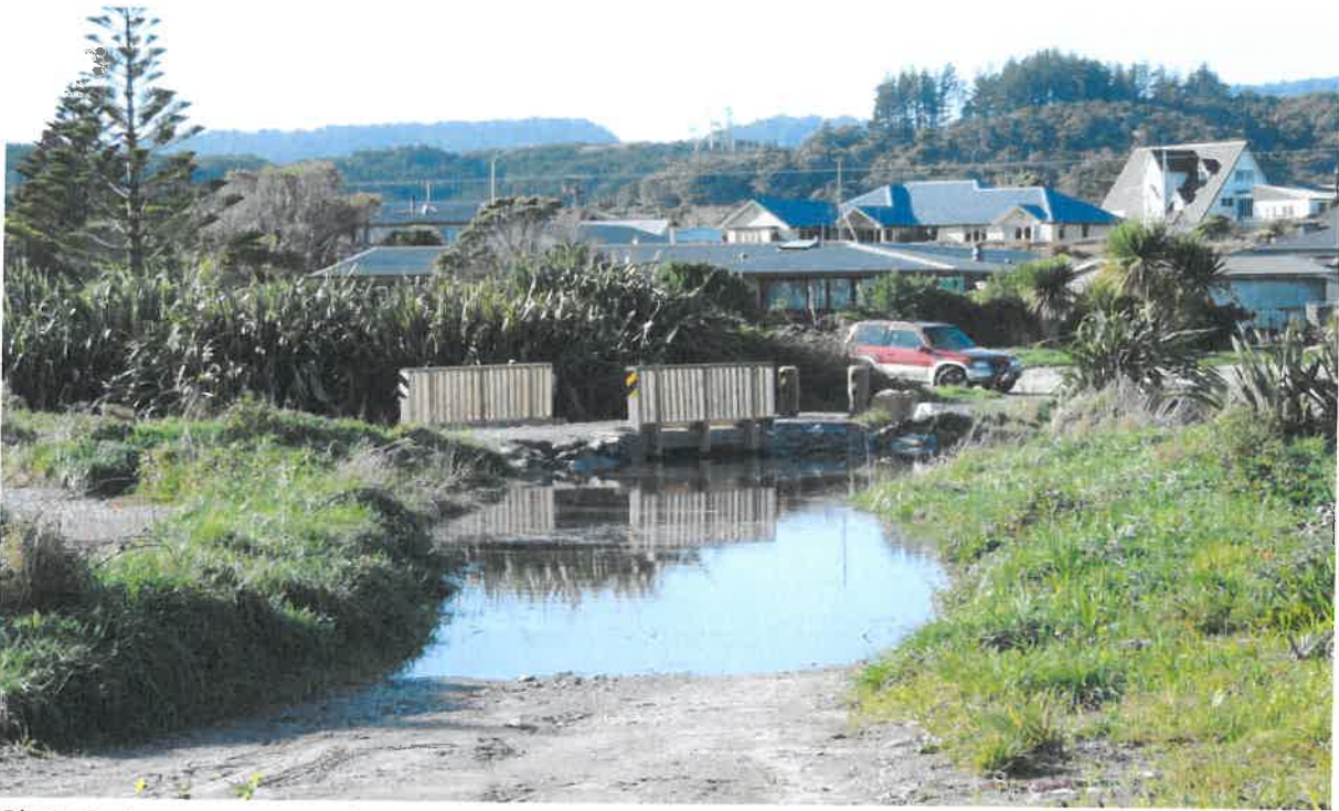
Photo 1: Cycle-way bridge before opening
