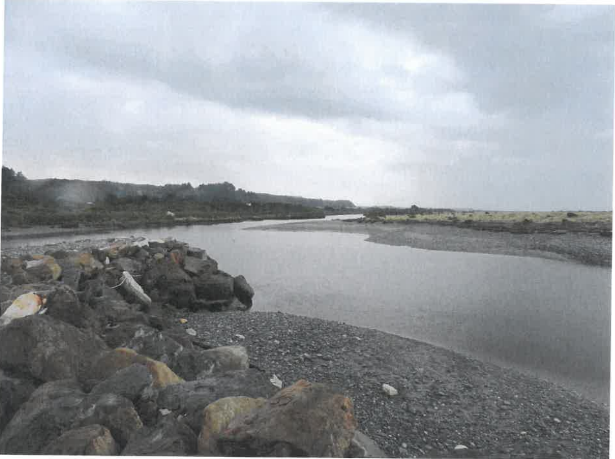
Photo 4: New River 18 hours after outlet opened.
