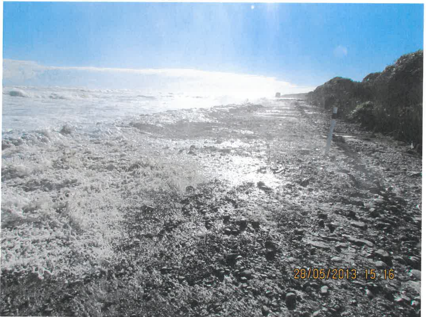
Punakaiki Rating District Seawall – Overtopping by Wave Action – King Tide 28 May 2013
