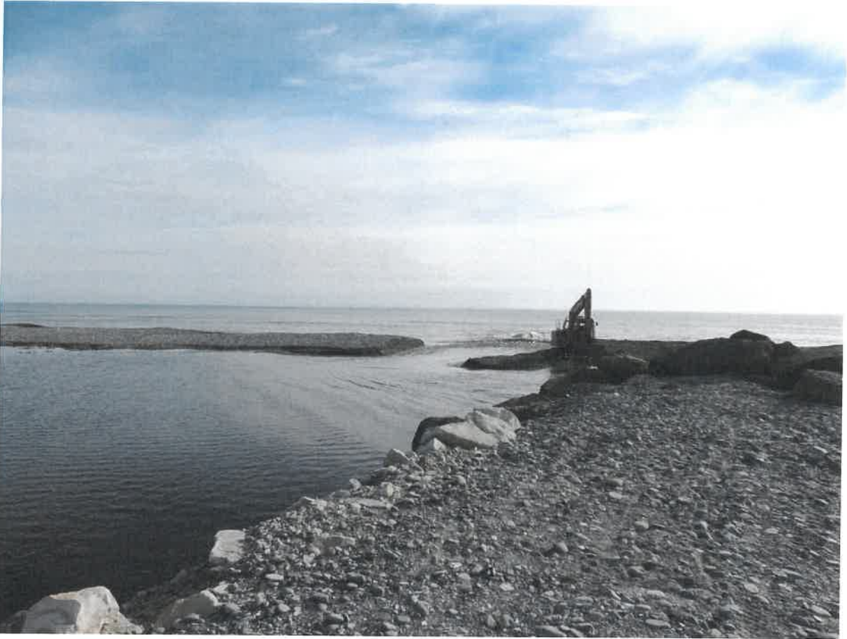
Photo 5: Westroads excavating outlet
