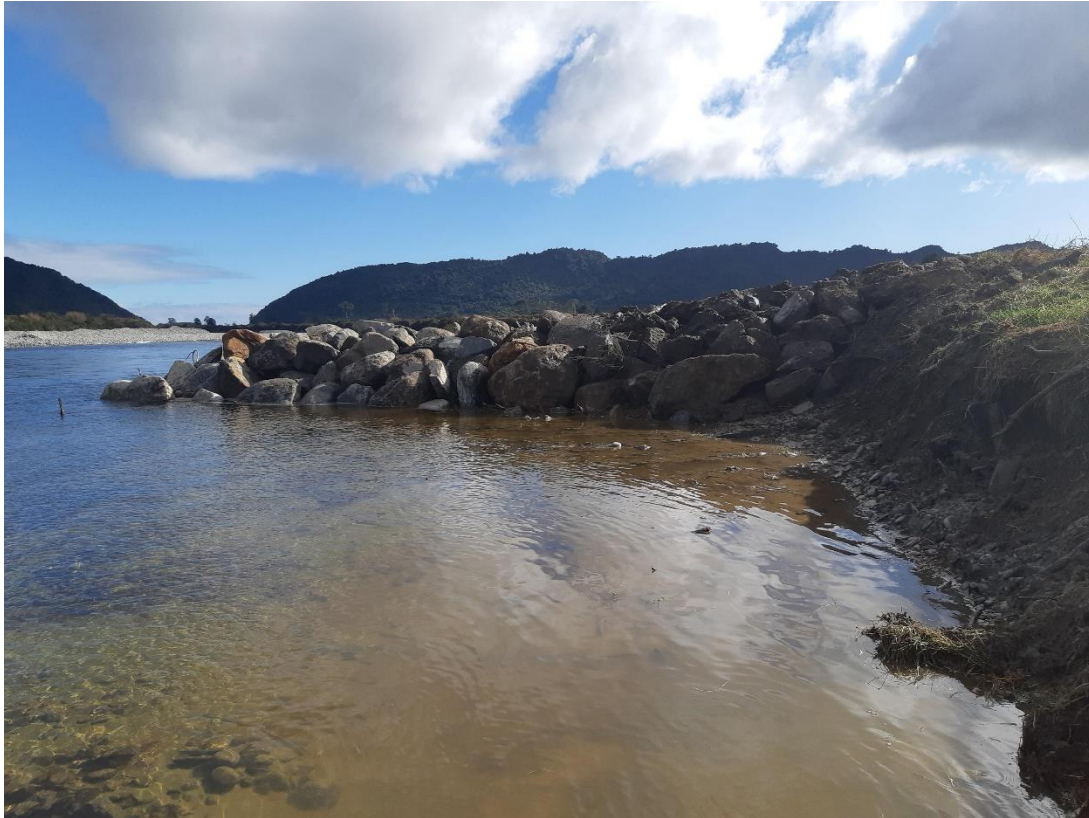
Extended spur directly upstream of the diversion cut at Omoto.
