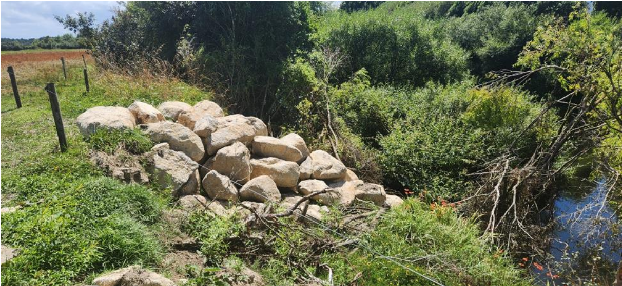
Repaired Nikau Farm spurs.
