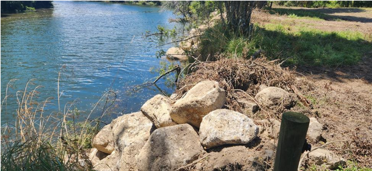
Glasseye Road rock spurs and scrub clearance.
