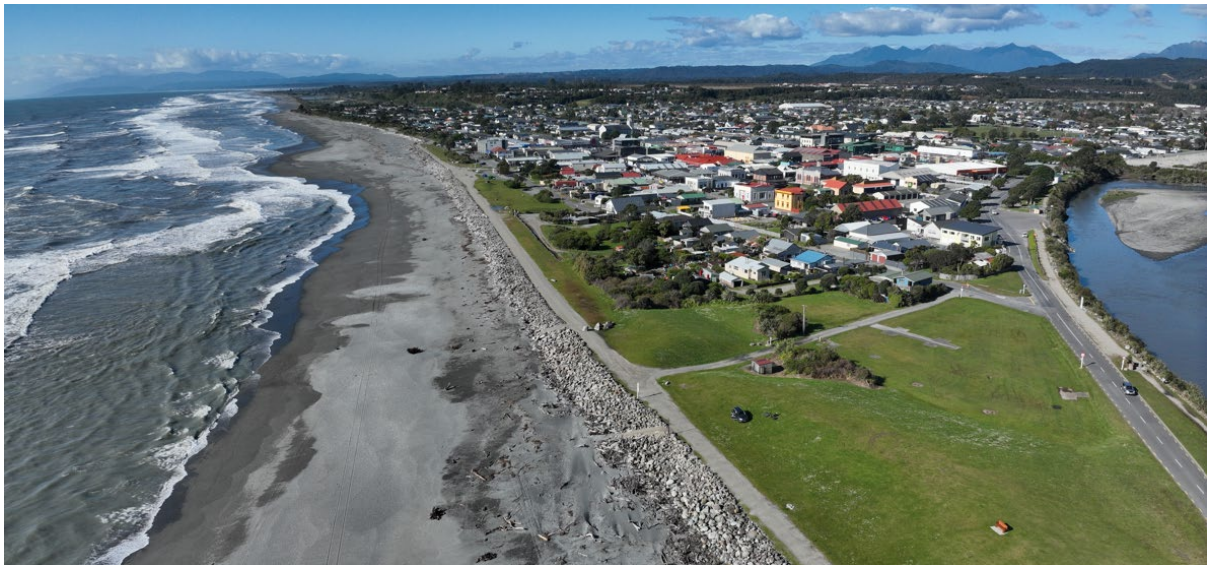
Figure 5: View of the Hokitika Seawall looking north toward Richards Drive
