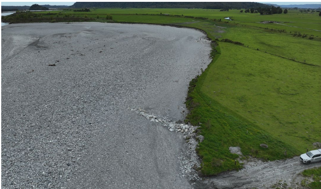
Figure 4: View of the lower retards looking downstream following the October rainfall events
