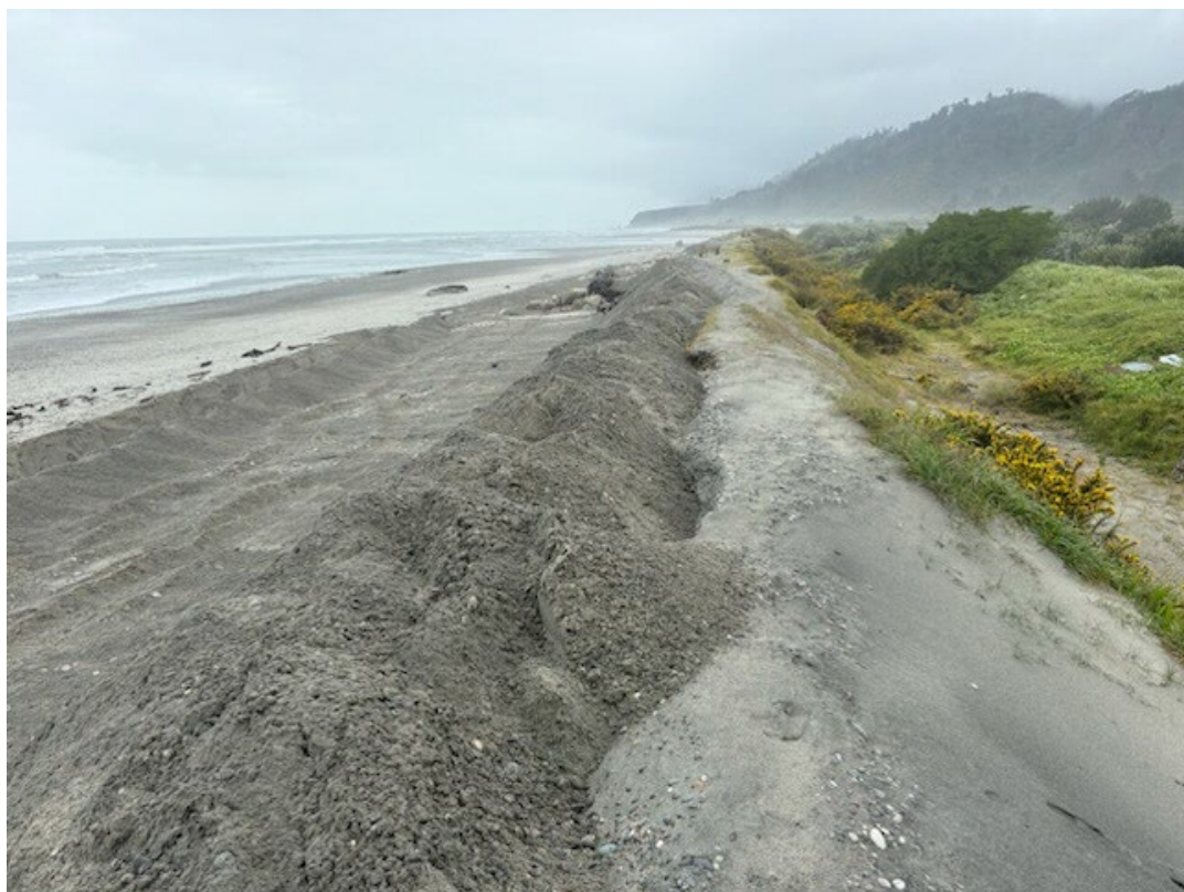
Figure 2: Replenished sacrificial seawall
