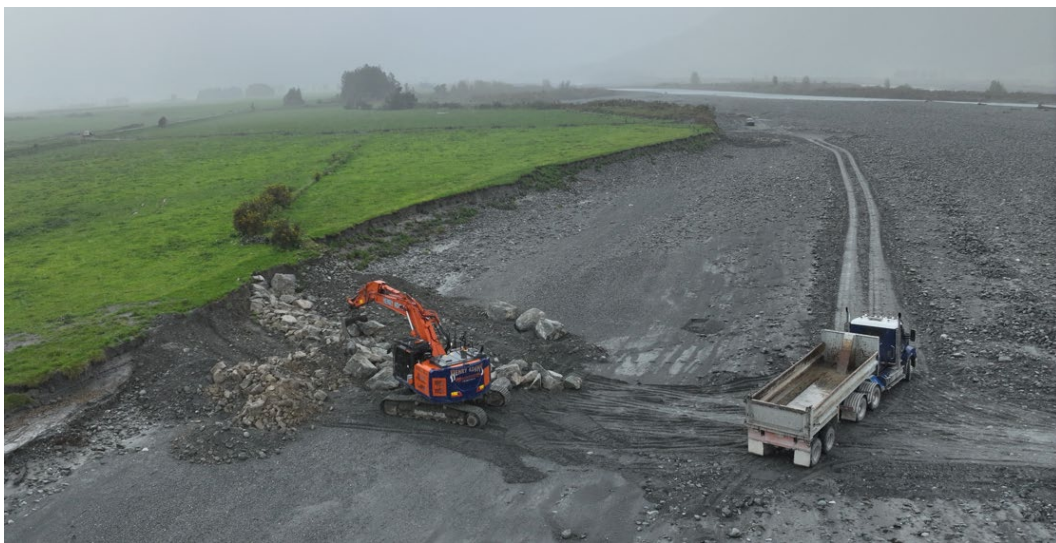
Figure 3: Construction of the middle retard in progress
