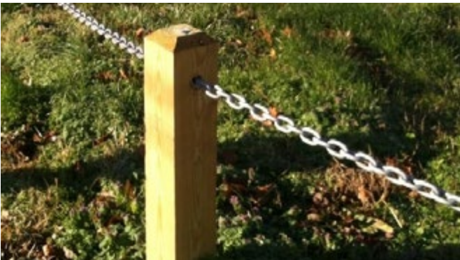
Fencing Typology 2 - Post and Chain Access Gate with lock
