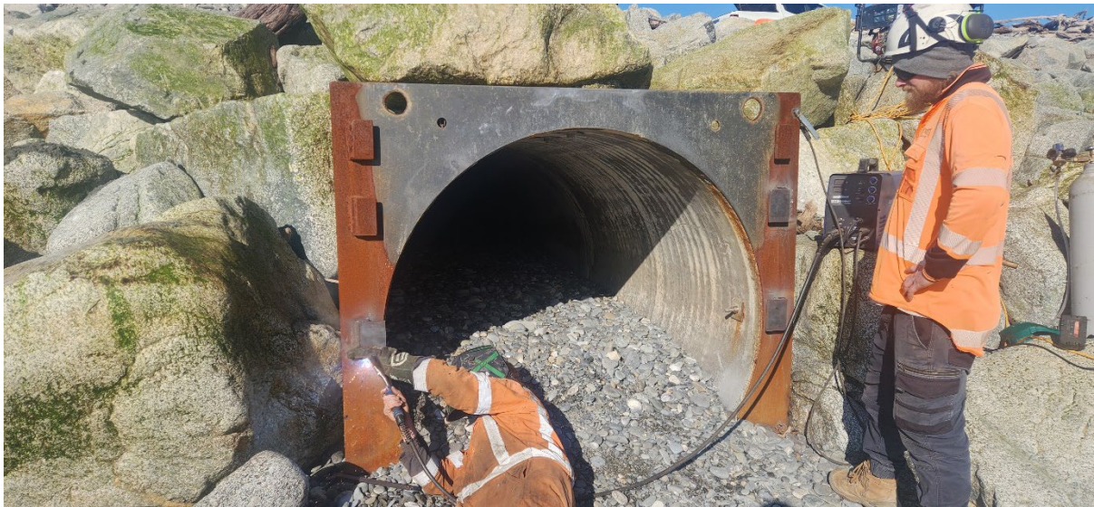
Repairing the guides.
