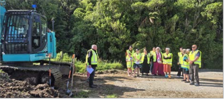
Flood protection Recovery work in Westport (Photo credit: Resilient Westport)
