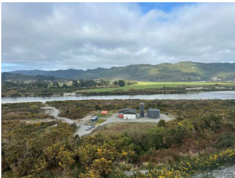
Figure 5: Grey District Council's water treatment plant
