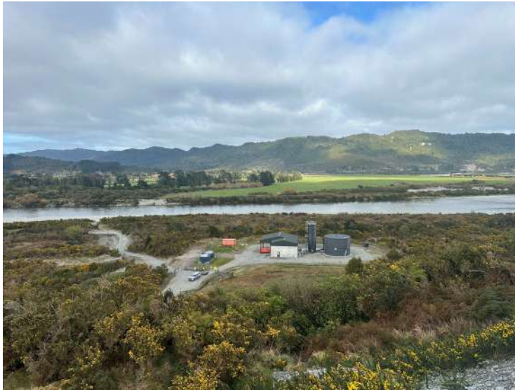
Figure 5: Grey District Council's water treatment plant
