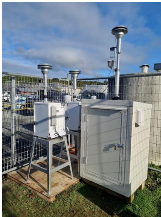
Figure 73. Monitoring equipment at the Greymouth High School site, winter 2025.
