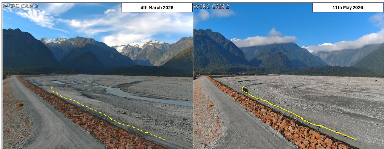
Figure 8 - Lateral erosion at the upstream end of Havill's Wall over a two month period.
