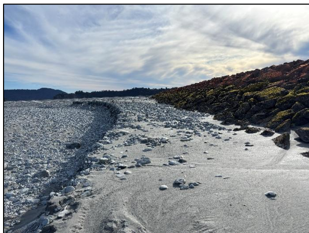
(c) 20 – 50 m buffer remaining between channel and a section of Havill's Wall
