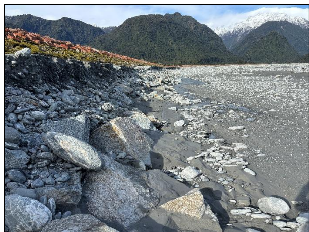
(b) Exposed stopbank toe at the downstream end of Havill's Wall.
