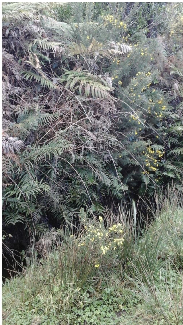
Figure 51 Looking into the western end of the designation showing the drain
