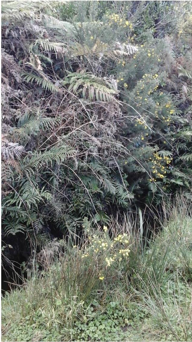
Figure 51 Looking into the western end of the designation showing the drain
