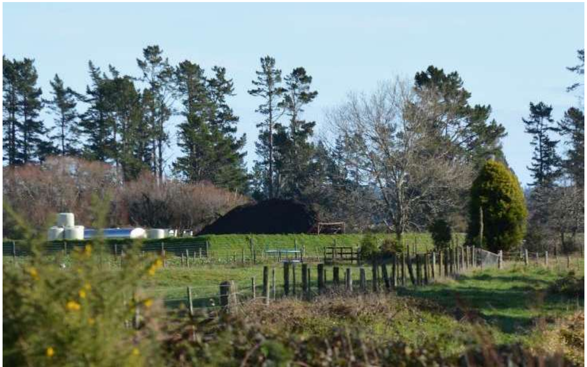
The stockpile of fly ash on site as seen from the Kokatahi Kowhitirangi School on Upper Kokatahi Road above the constructed bund.
