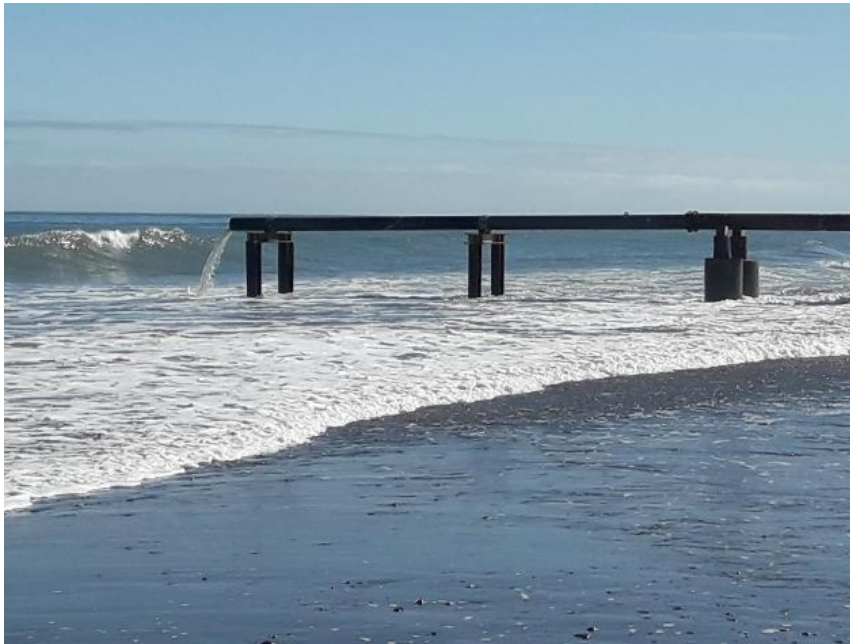
Figure 3-9: The existing WDC wastewater outfall at the Hokitika coastline
