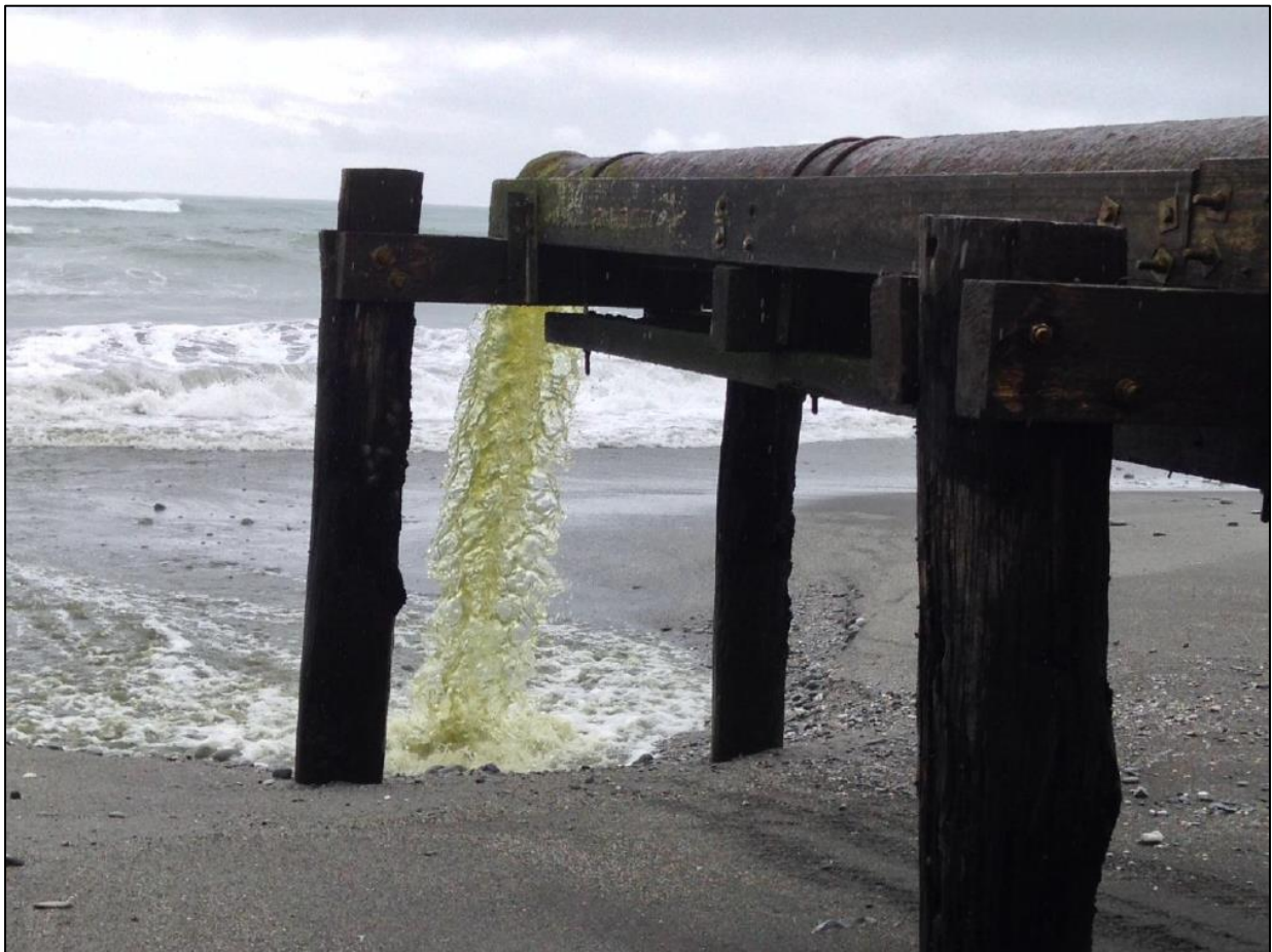
Figure 2: Photo of discharge via outfall at low tide (source: Riverlake, 2015)
