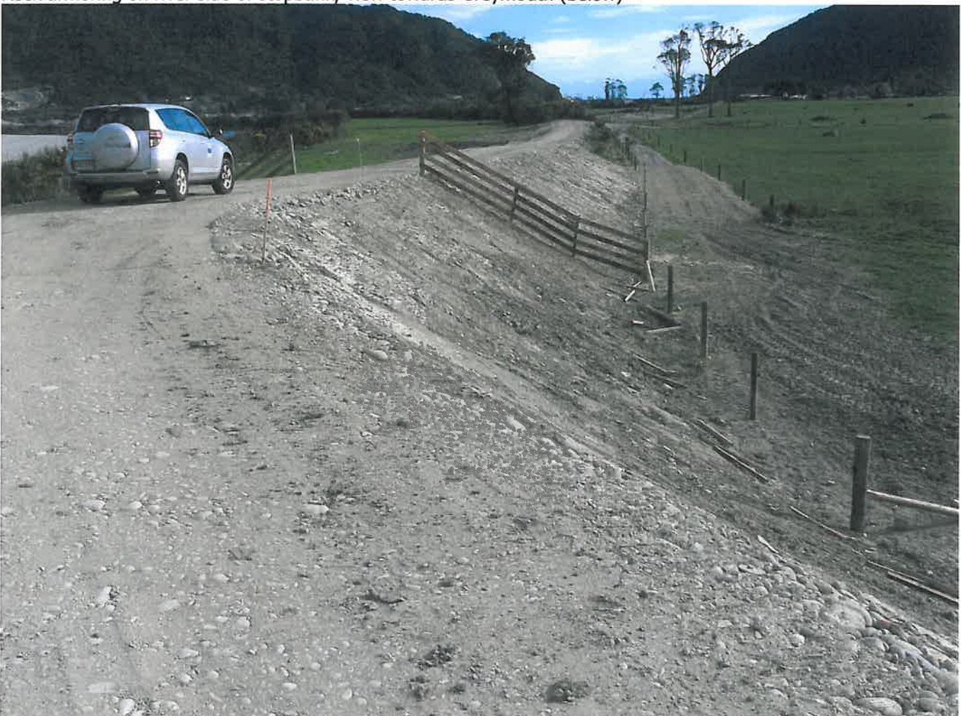
Rock armoring on river side of stopbank, view towards Greymouth (below)
