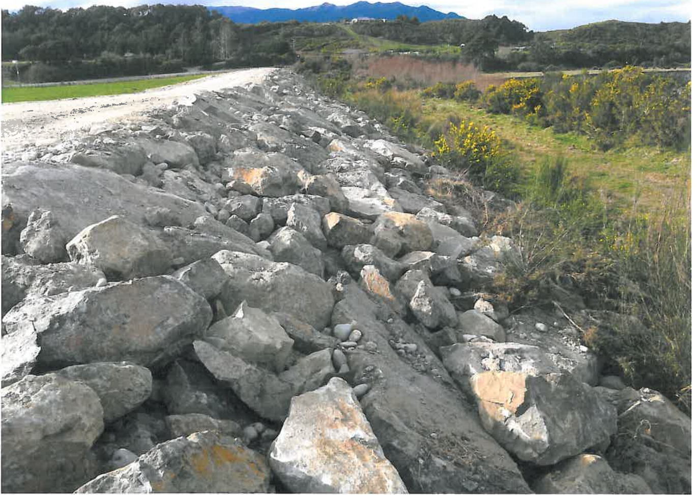
Rock armoring on river side of stopbank, view towards Greymouth (below)
