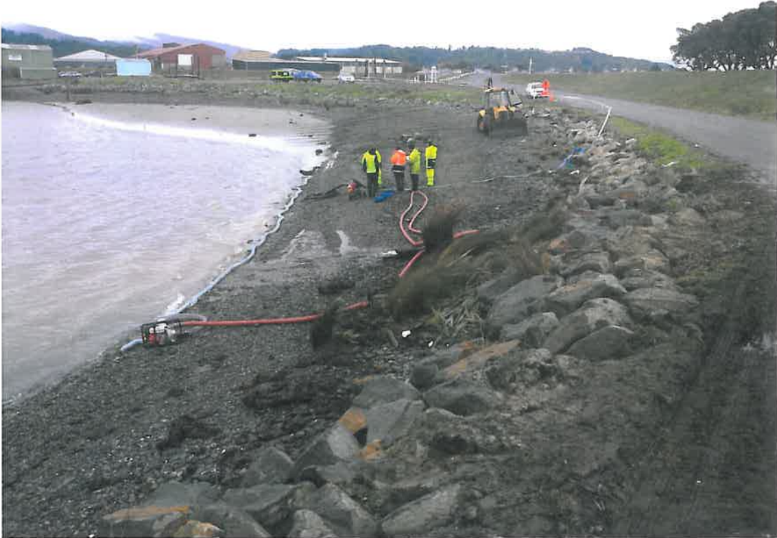
Pumps and absorbent booms deployed
