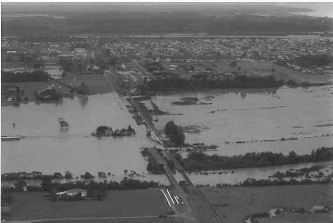
Stephen Road bridge over the Orowaiti River near Sergeants Hill
