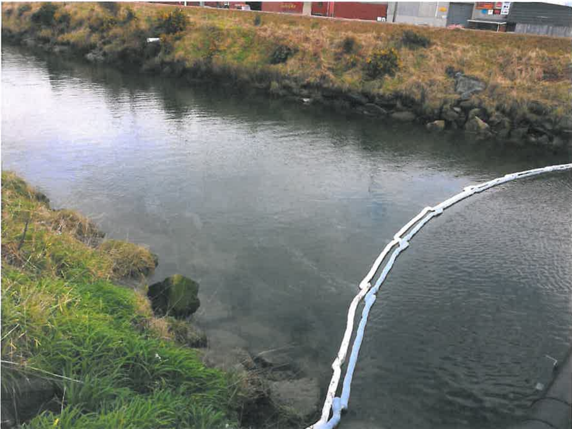
Inlet to the lagoon protected with absorbent booms
