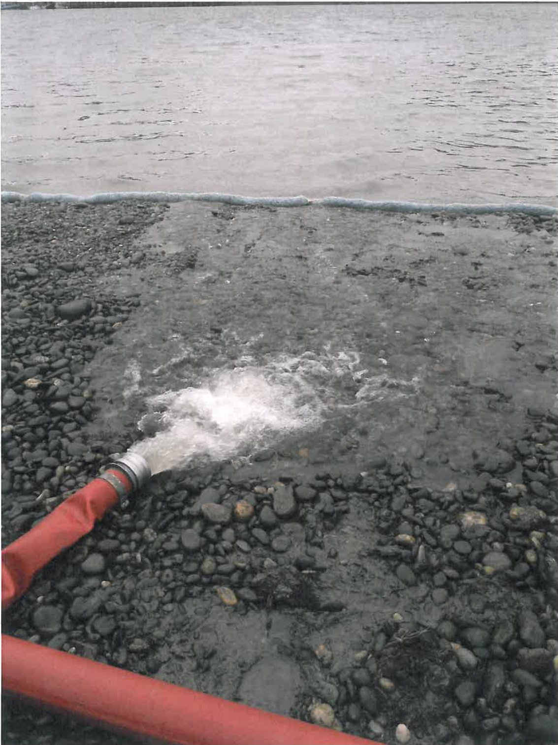
Pumping operation to direct diesel on foreshore towards the absorbent booms
