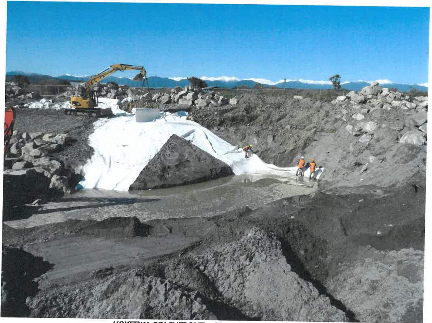
HOKITIKA BEACHFRONT – 29 August 2013 South End Showing Placing of Filter Fabric
