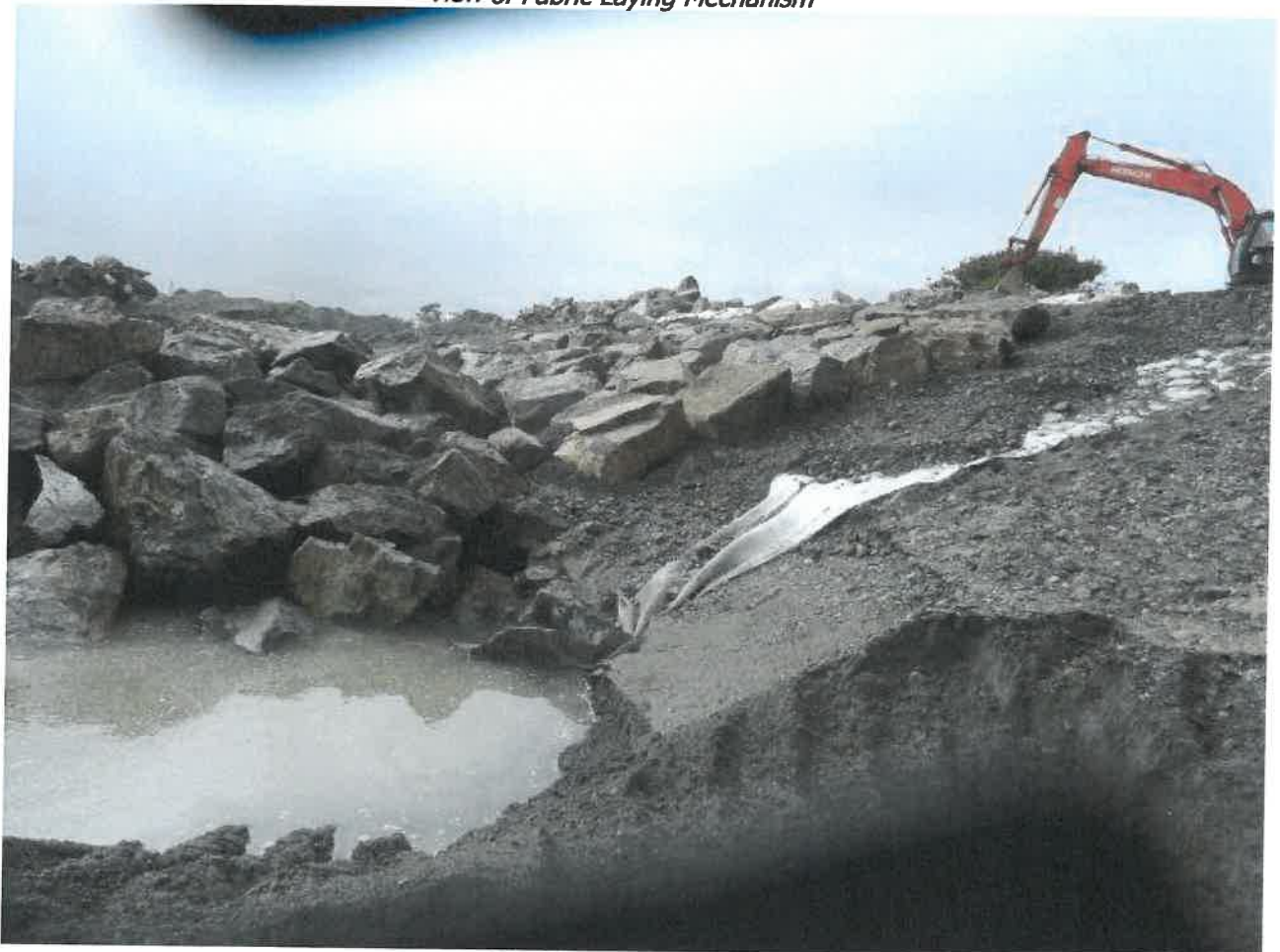
HOKITIKA BEACHFRONT – 27 August 2013 Placing of 1 st layer of Heavy Rock Armouring
