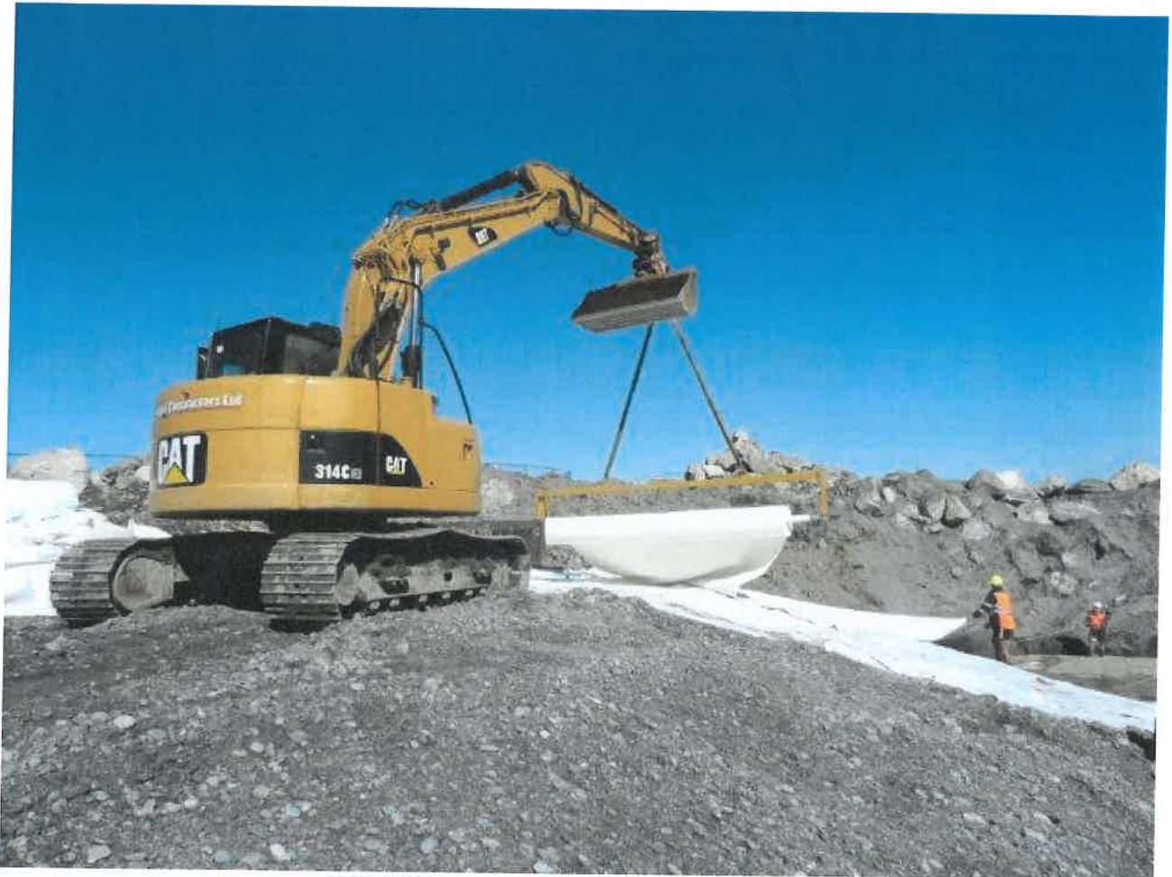
HOKITIKA BEACHFRONT – 29 August 2013 View of Fabric Laying Mechanism
