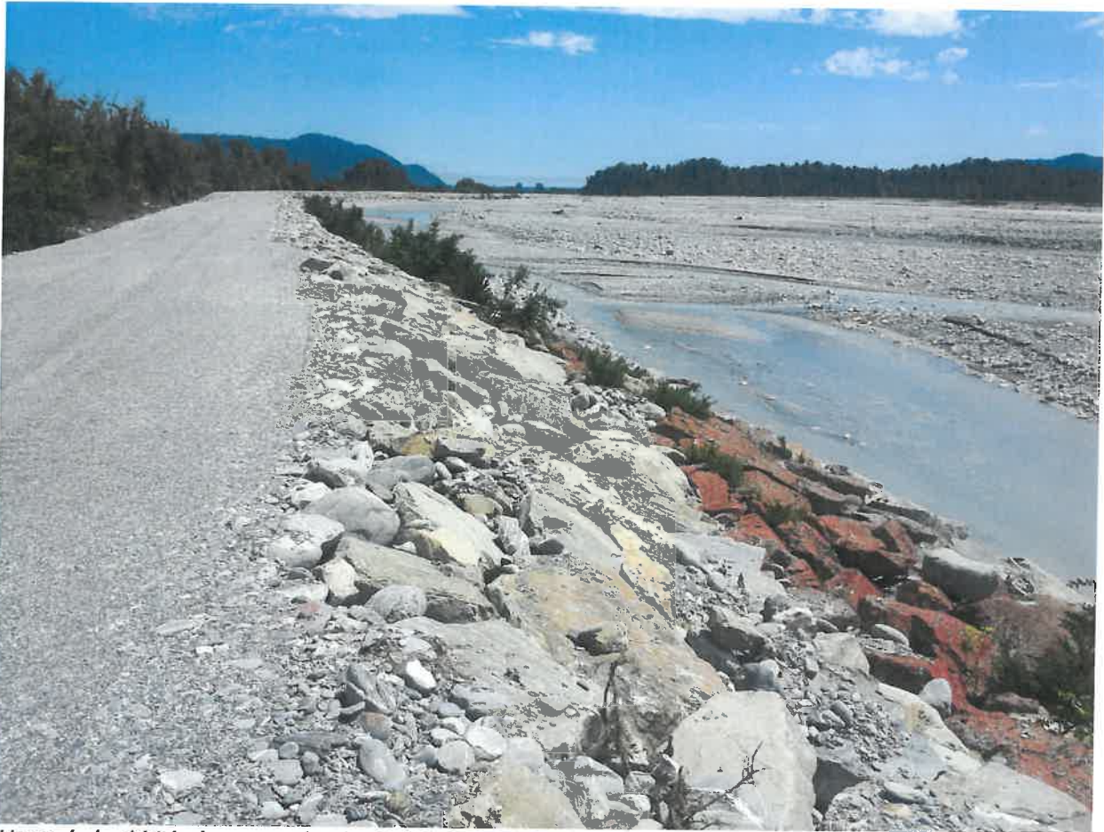
Upgraded rubbish dump stopbank looking downstream
