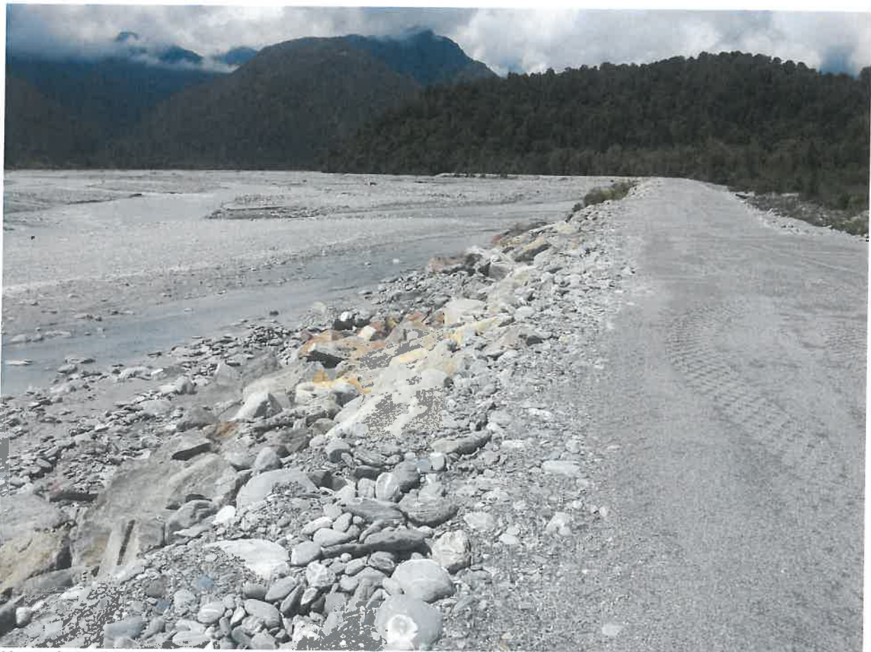
Upgraded rubbish dump stopbank looking upstream
