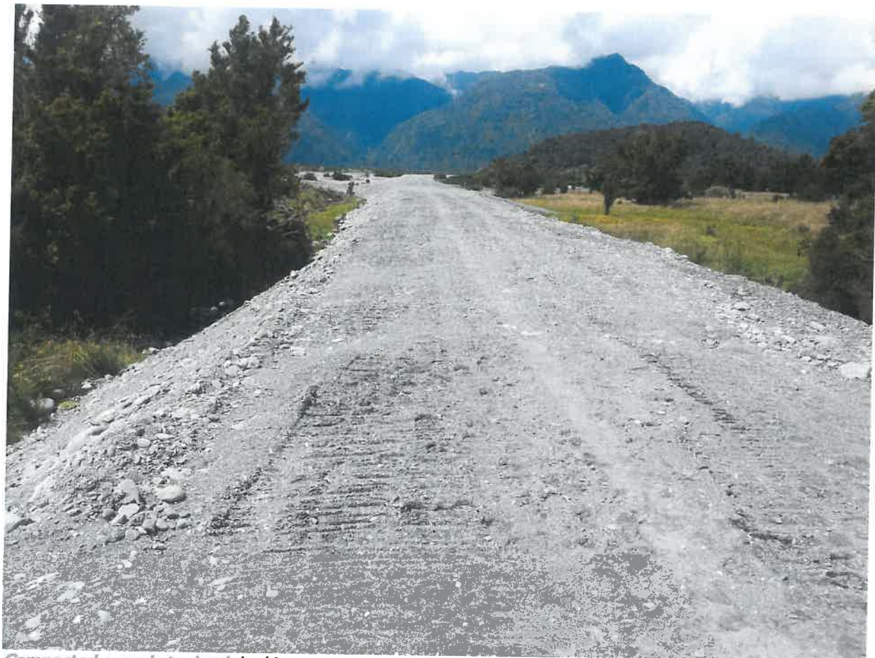
Compacted gravel stopbank looking upstream towards rubbish dump stopbank
