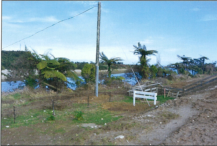
New telecommunications pole and wire stay alongside stopbank, 19 July 2017.
