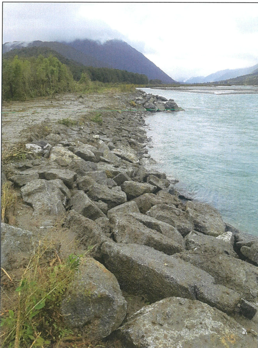
Completed rock Riprap between existing Groynes
