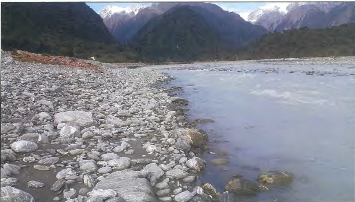
15 May 2018 Monitoring – River training looking upstream
