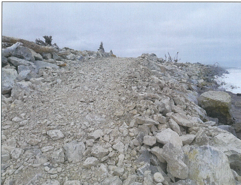
Repair of access ramp.
