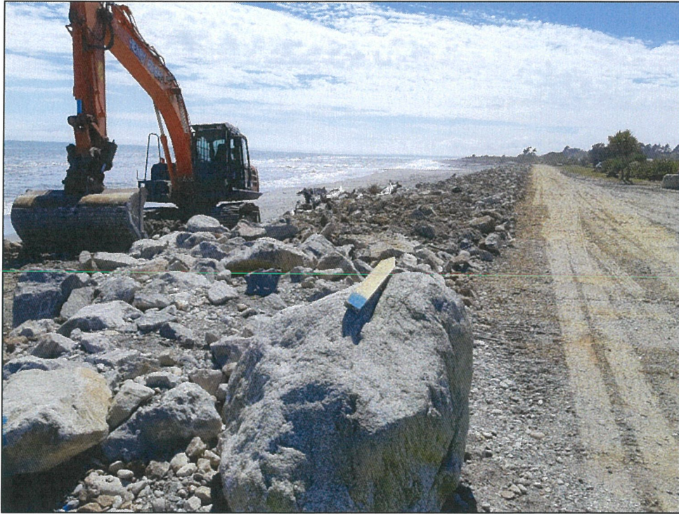
Top up of slumped areas on top of the seawall.
