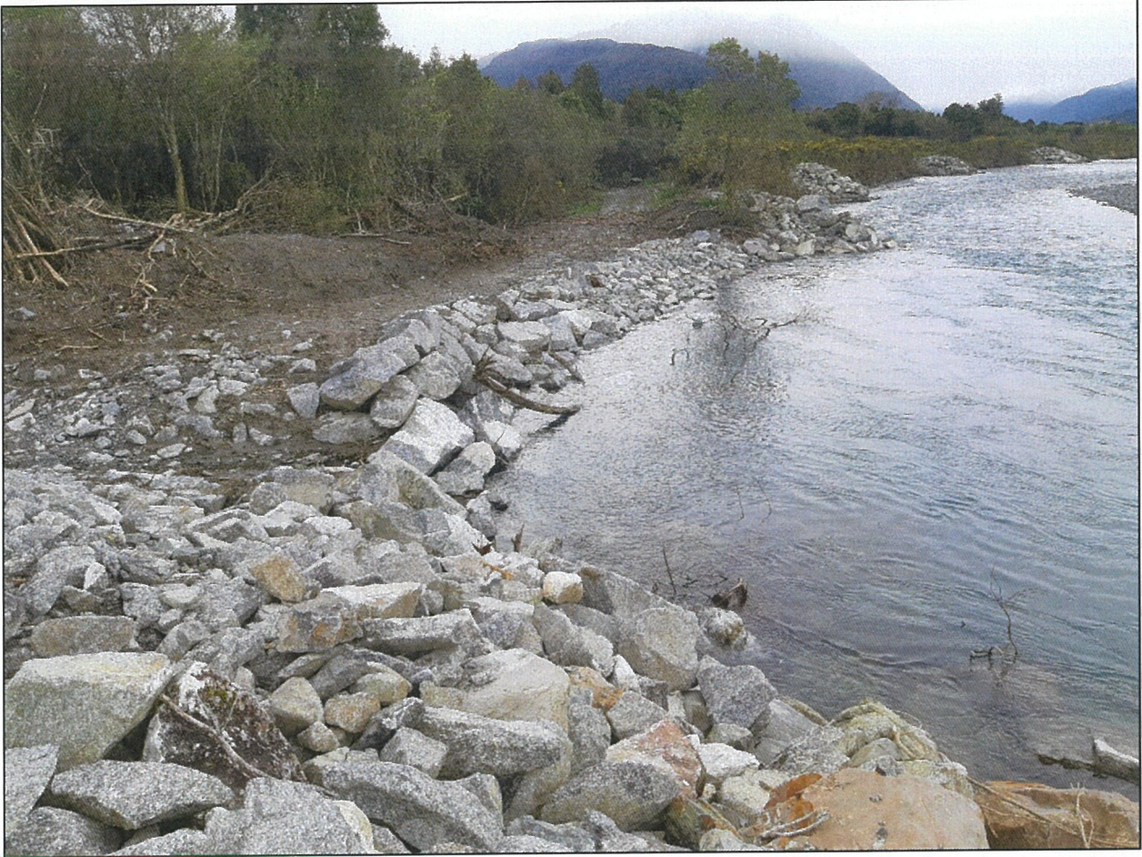
Completed riprap rock work
