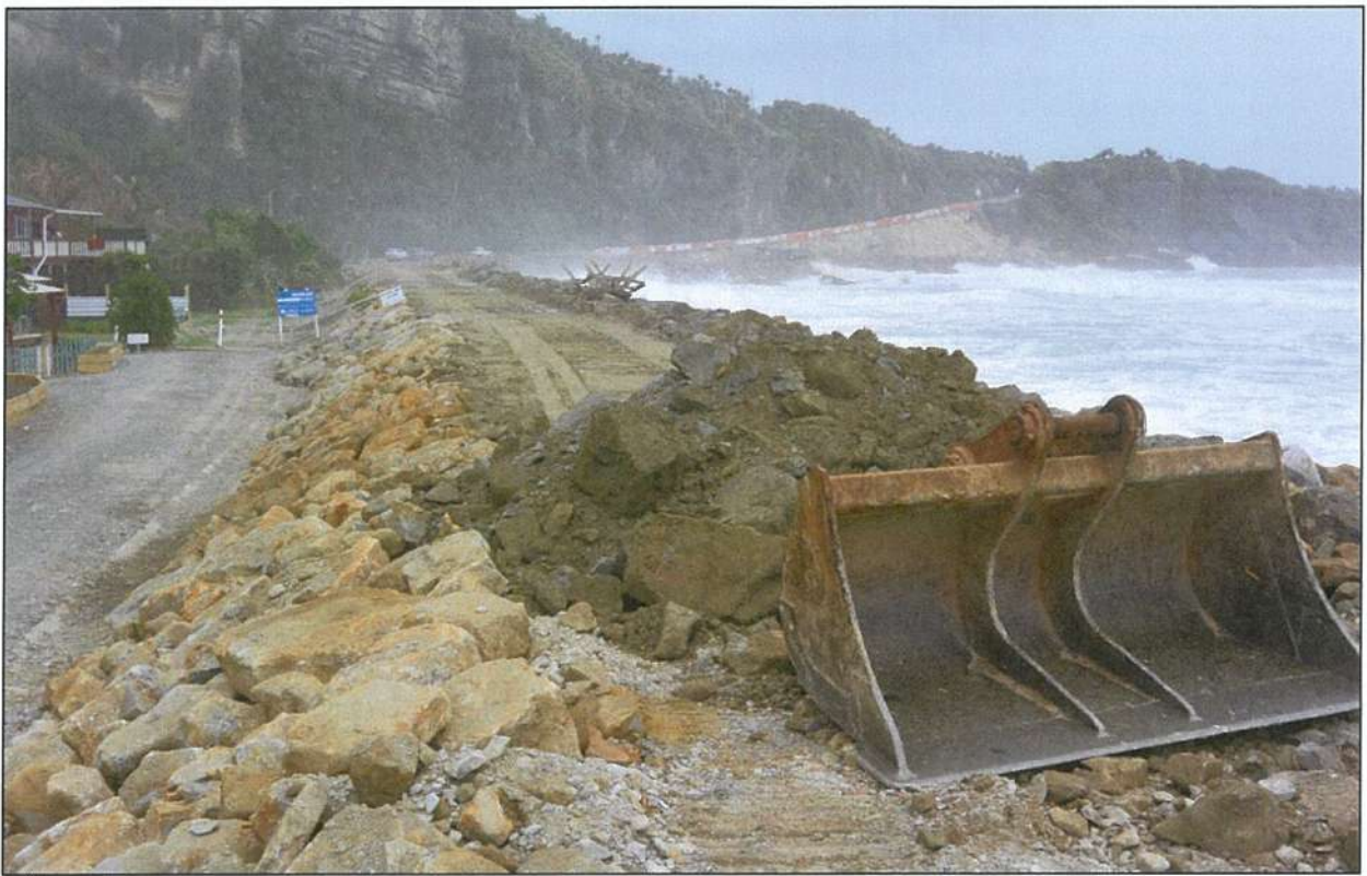
Looking south. Crest reformed and placement of riprap.
