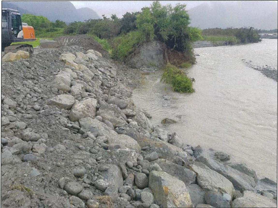
View of repair of stopbank underway
