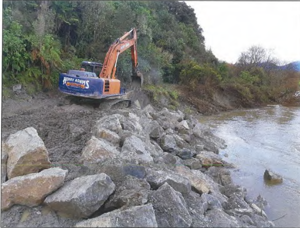
Repair Works under construction
