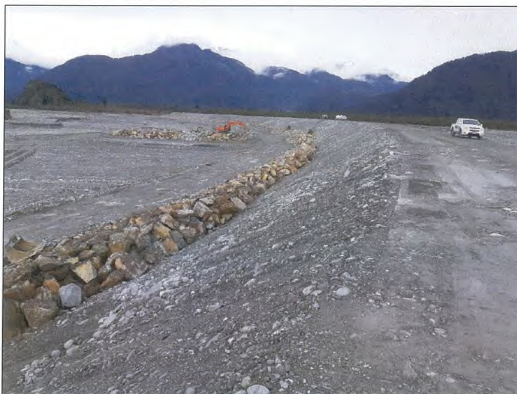
Completed section of new Stopbank – with rock placed to half height
