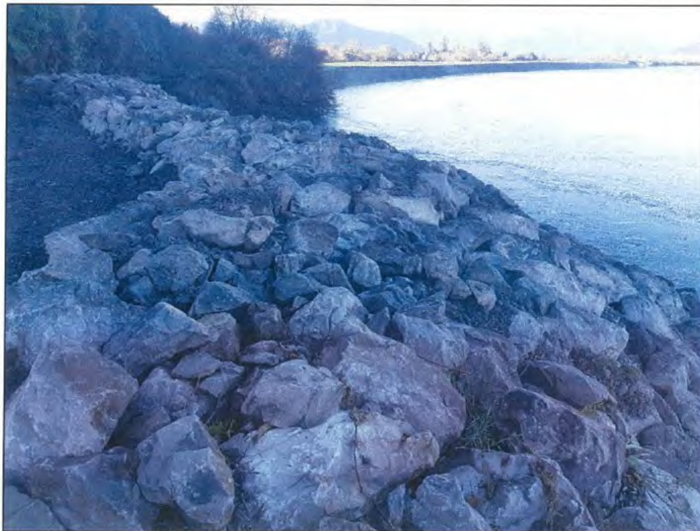
Completed repair works
