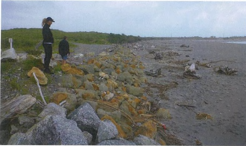
Figure 3-2: Rock extension south of the carpark to protect the Lagoon Cut entrance. [Credit: M. Hicks, 21/11/2017].
