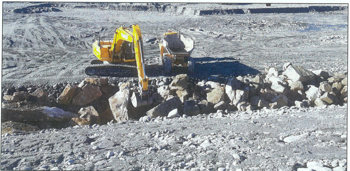
Completed section of new Stopbank – with rock placed to half height
