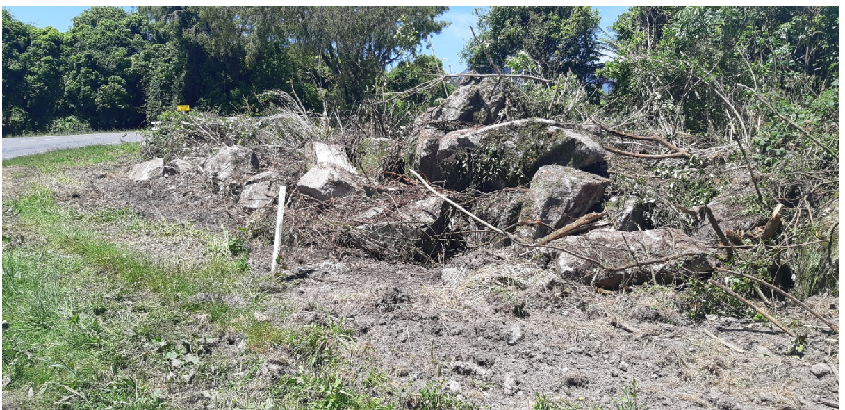
Rock stockpile site cleared of vegetation.
