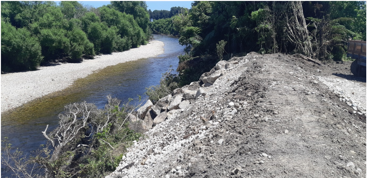
Looking downstream from the top of the rebuilt bank.
