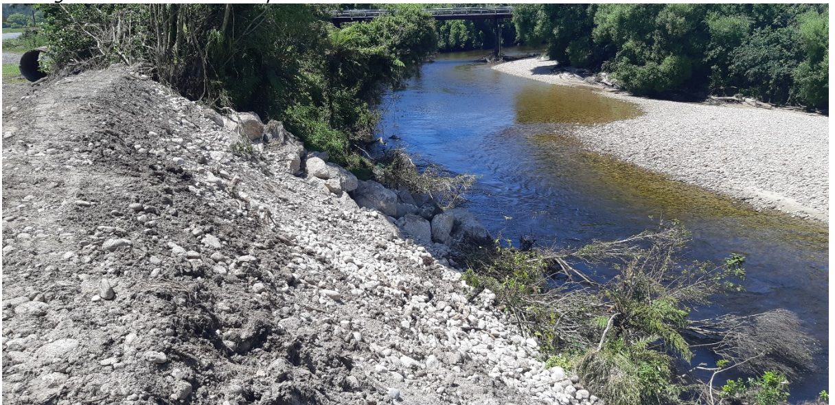
Looking upstream towards the road bridge.
