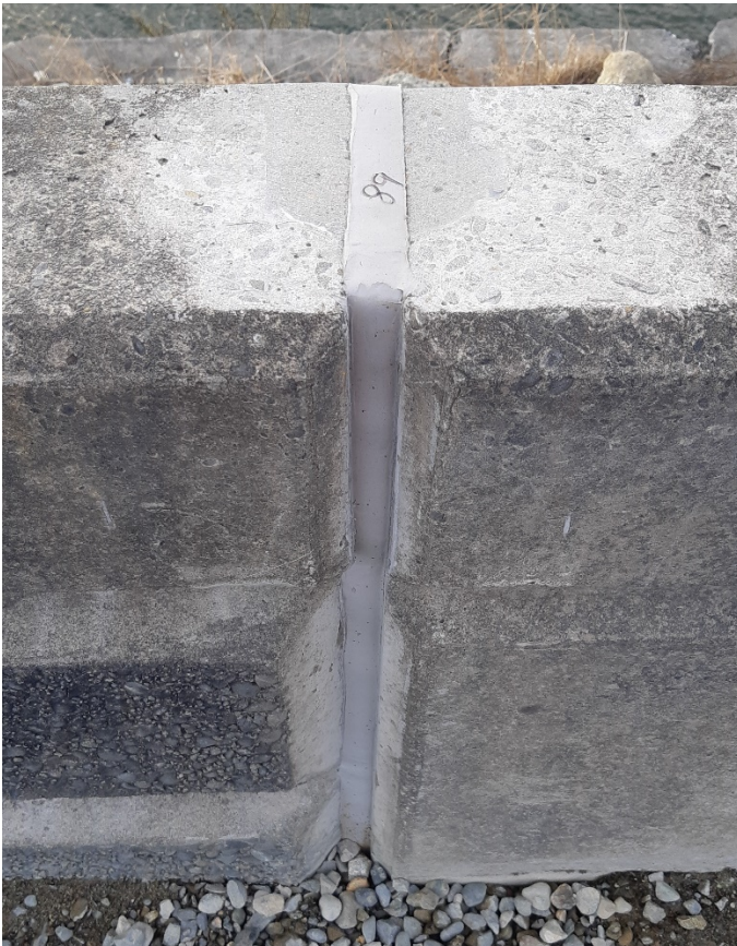
Example of a repaired and sealed joint.
