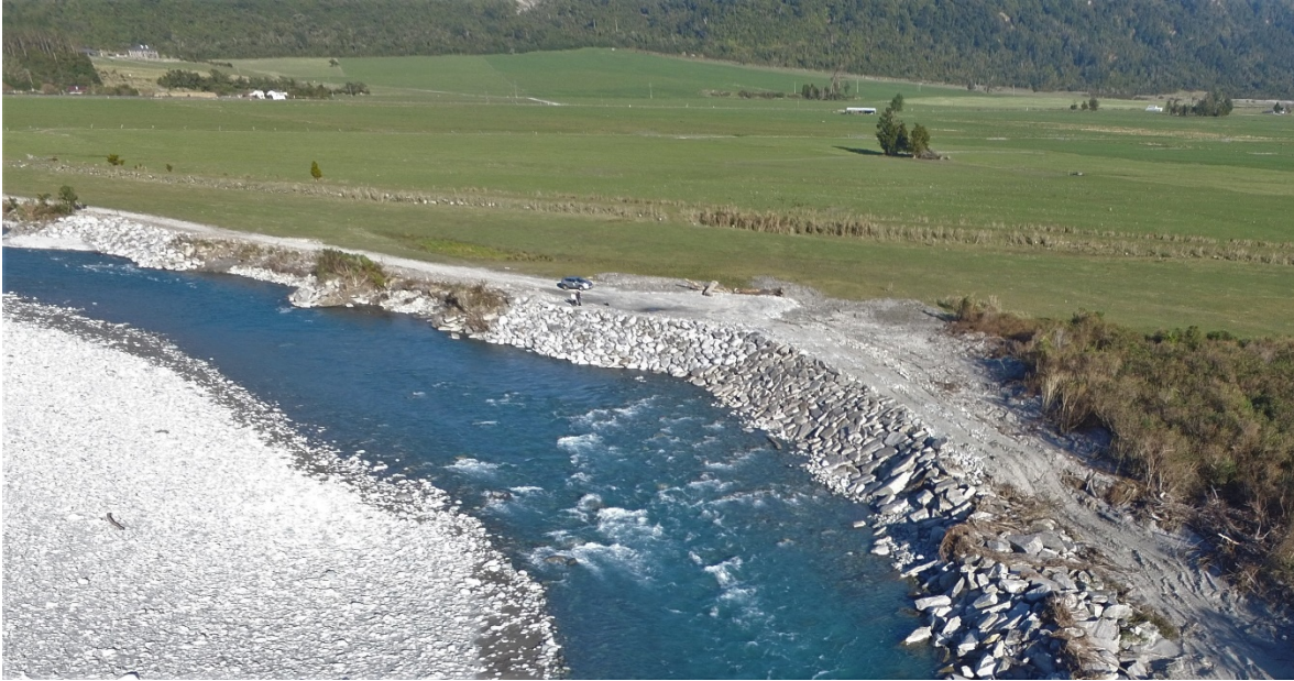
Drone image showing the completed work along John Sullivan's frontage.
