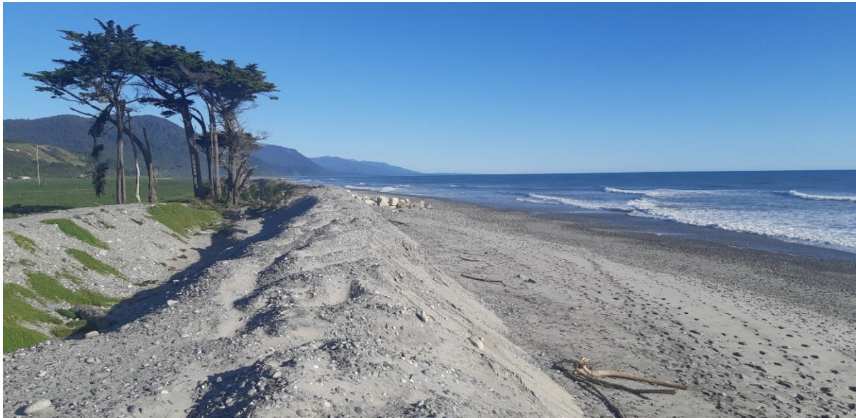
Looking south along crest of sacrificial wall.
