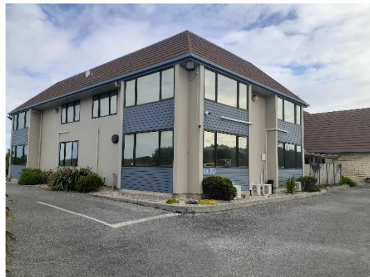
Photo 6 – View of side and front (south and east respectively) elevation of southern extension.
