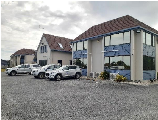
Photo 5 – View of rear and side (west and south respectively) elevation of southern extension.
