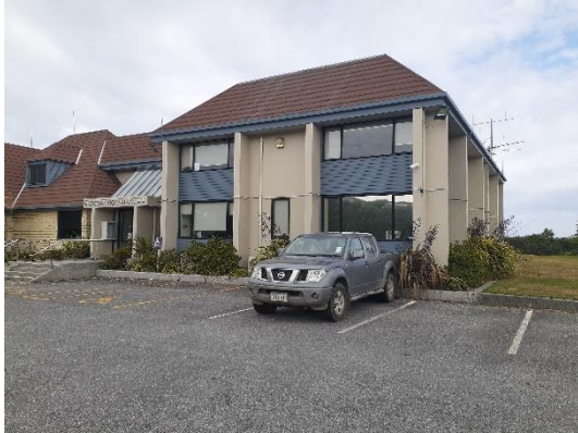
Photo 1 – View of front (eastern) elevation of Northern Extension
