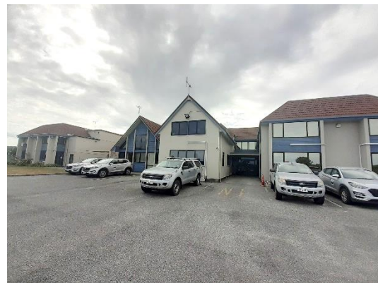
Photo 4 – View of rear (western) elevation of whole building.
