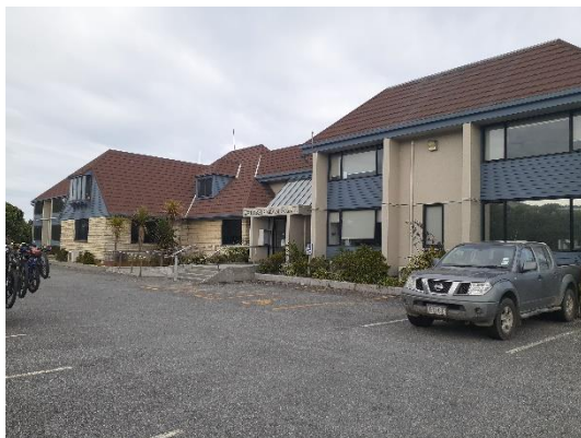
Photo 3 – View of front (eastern) elevation of whole building.
