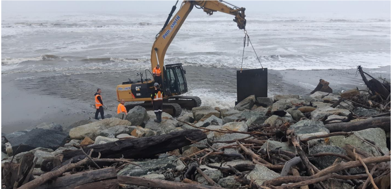
Photo 2. Removing the sliding gate
