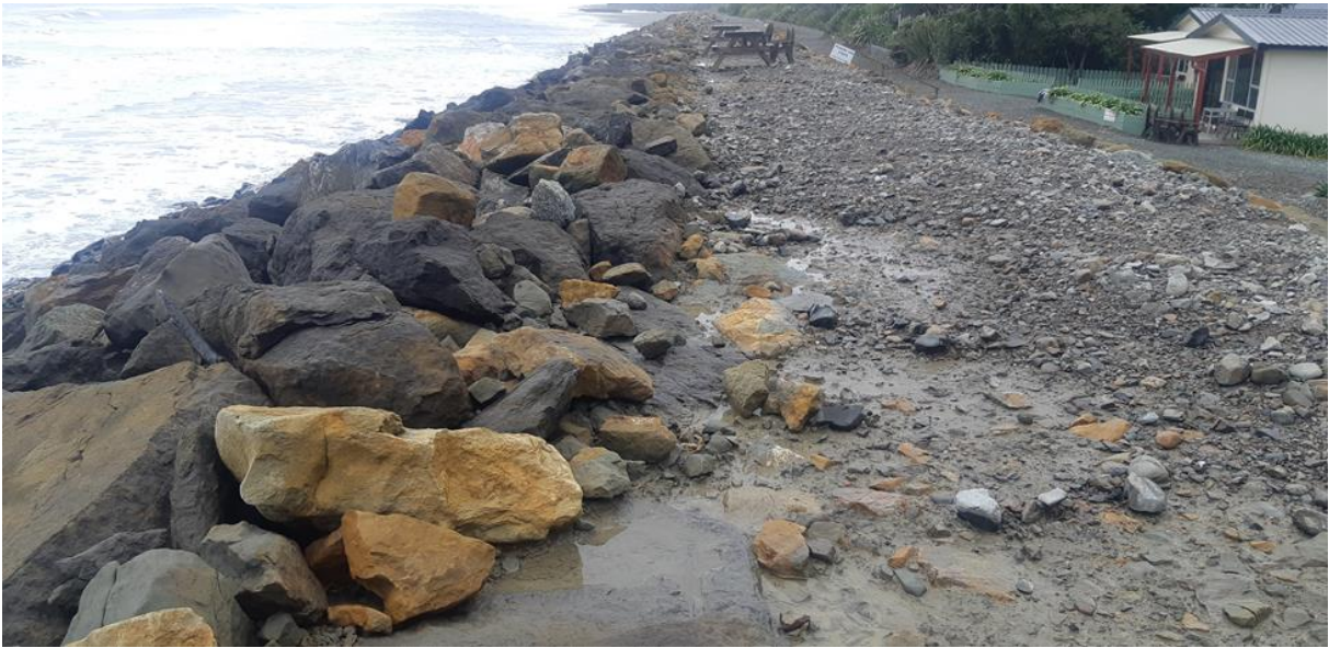
Punakaiki Seawall, looking north before start of works. May 2021
