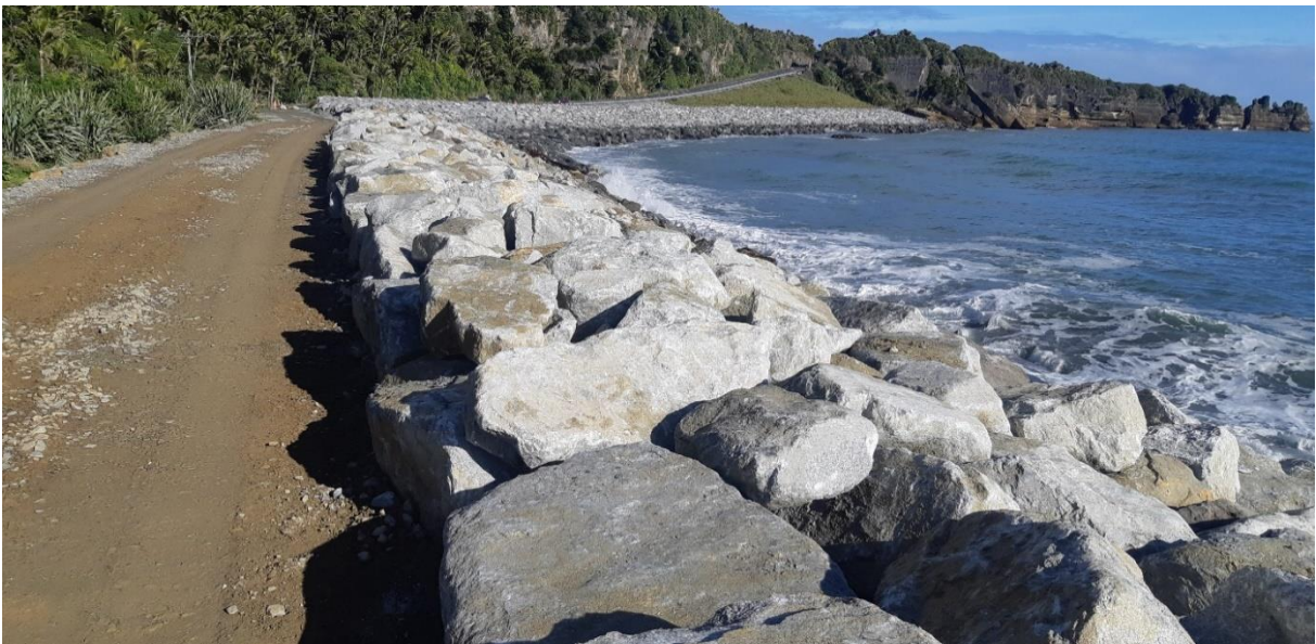
Punakaiki Seawall looking south, after works completed. July 2021
