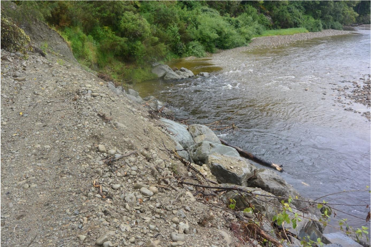
Photo 3. Erosion repair of upstream site
