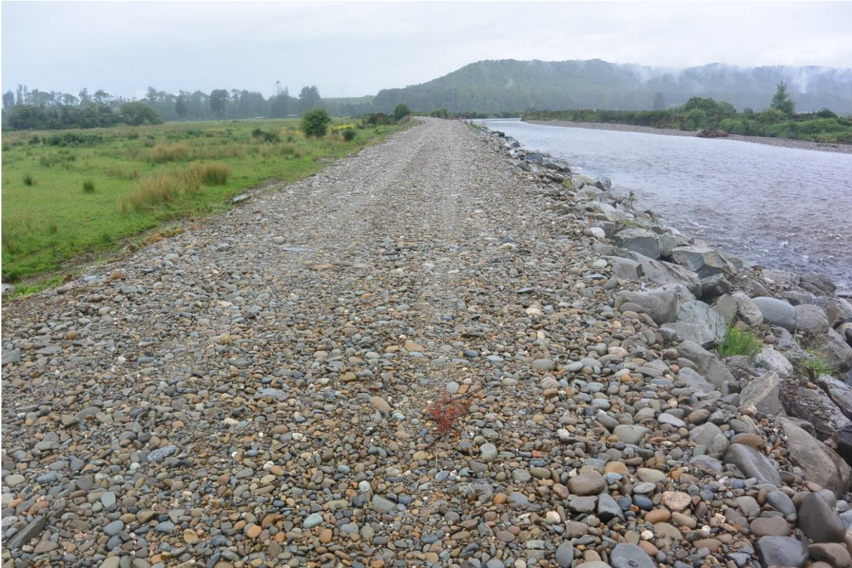
Photo 1. Looking upstream along stopbank crest
