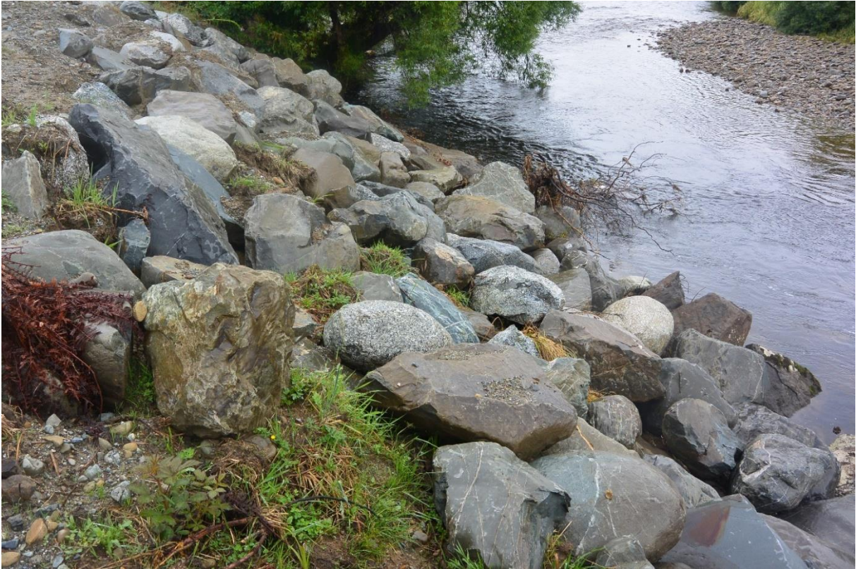
Photo 2. Repaired and riprapped stopbank
