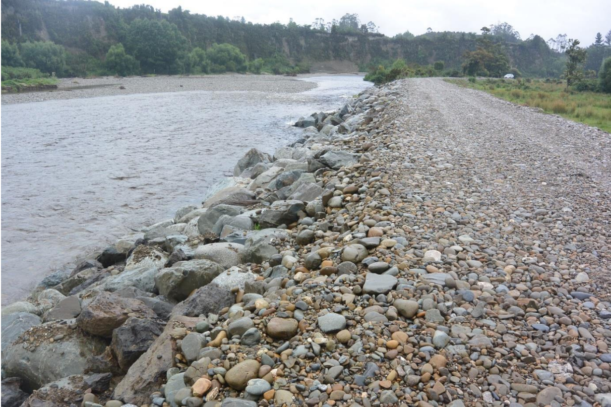
Photo 2. Looking downstream at repaired bank and rock spurs
