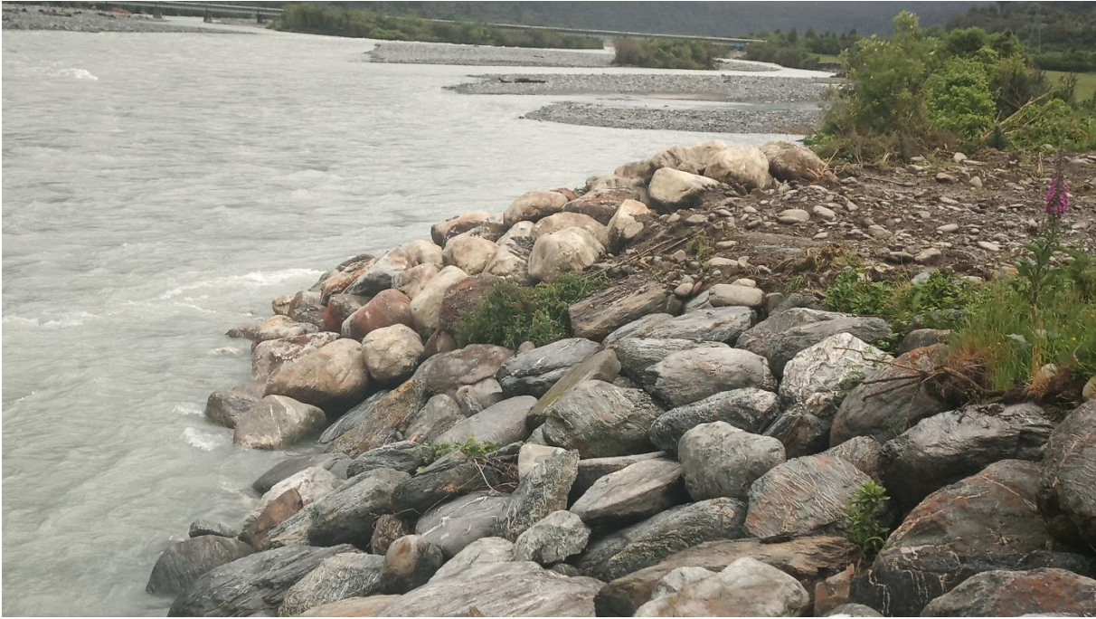
Repair to rock groyne at John Sullivan’s frontage
