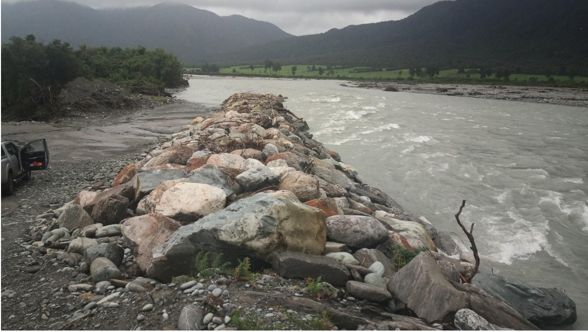
Repair to rock retard at John Sullivan's frontage
