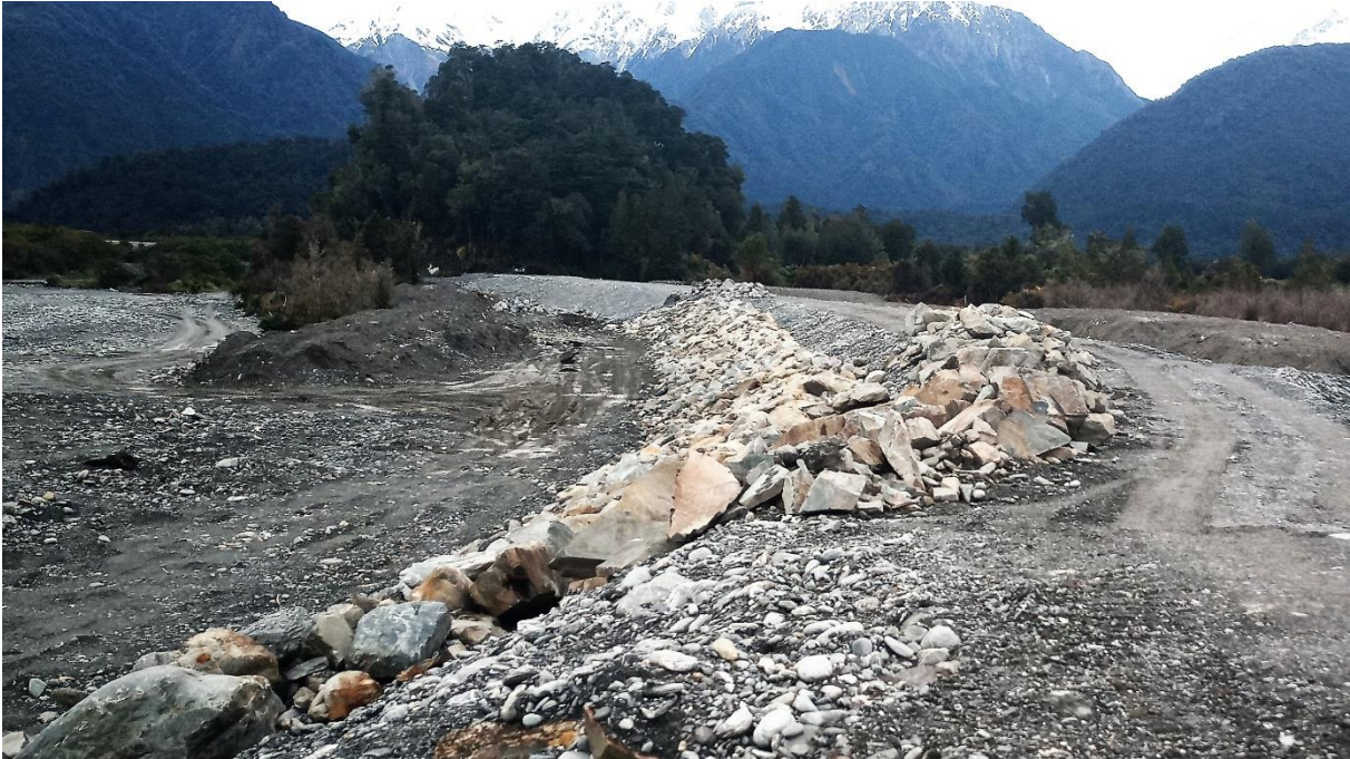
Looking up stream from Milton & Others Stopbank
