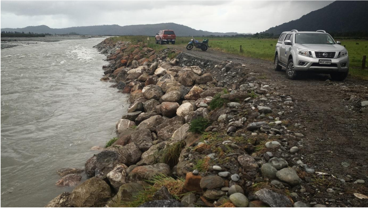
Rock work at Raymond Tuinier's frontage
