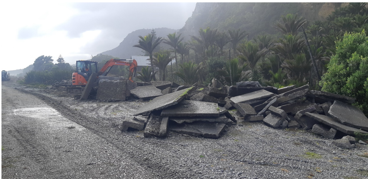
Digger heaping up the stockpiled blocks.
