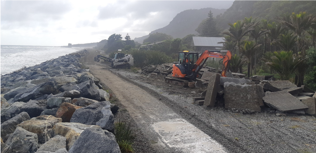
Crest of the seawall tidied up for pedestrians.
