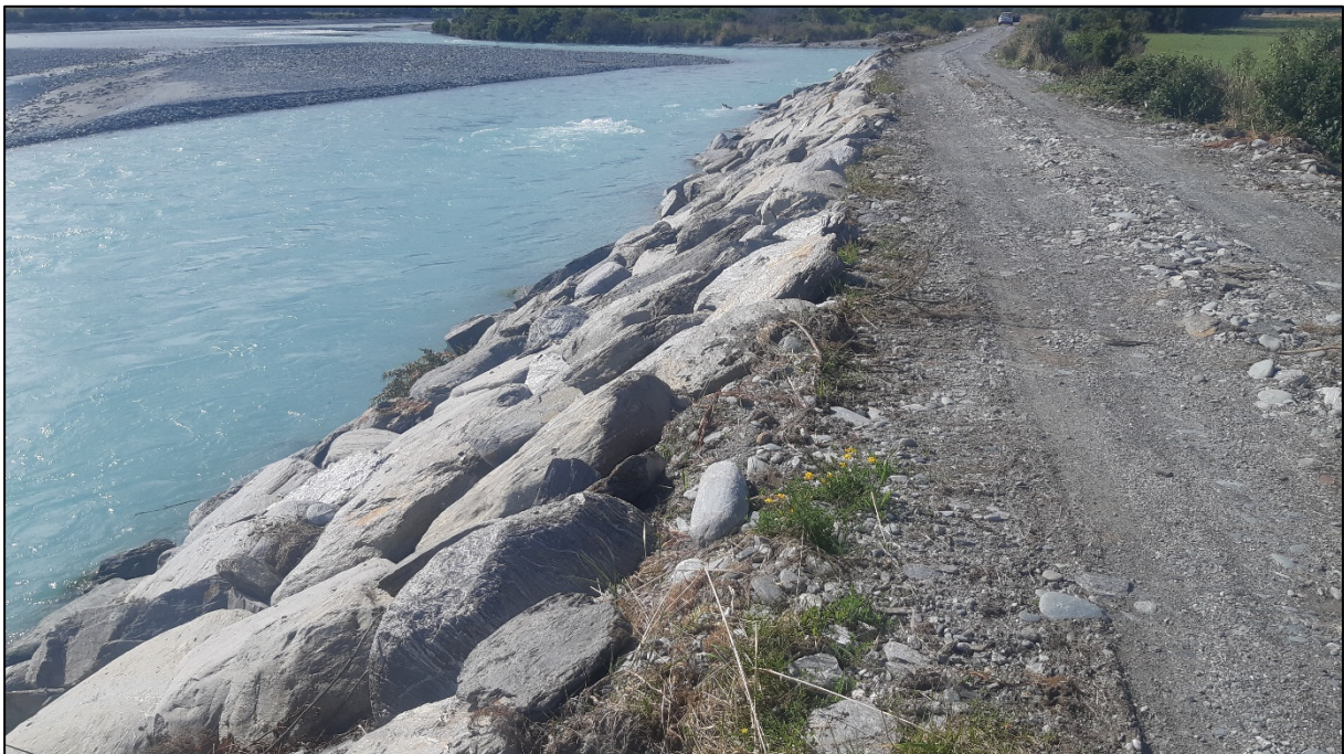
Completed maintenance work of rock riprap along Blackburn's Boundary Stopbank
