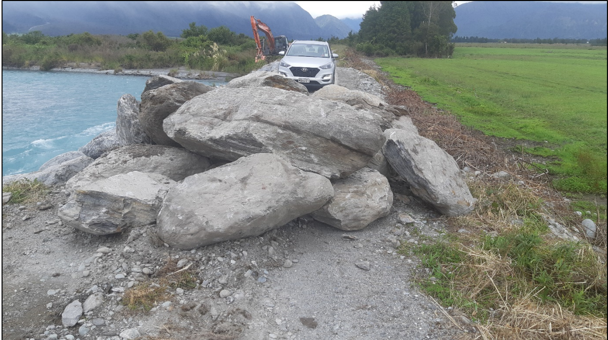
Rock ready to be placed
