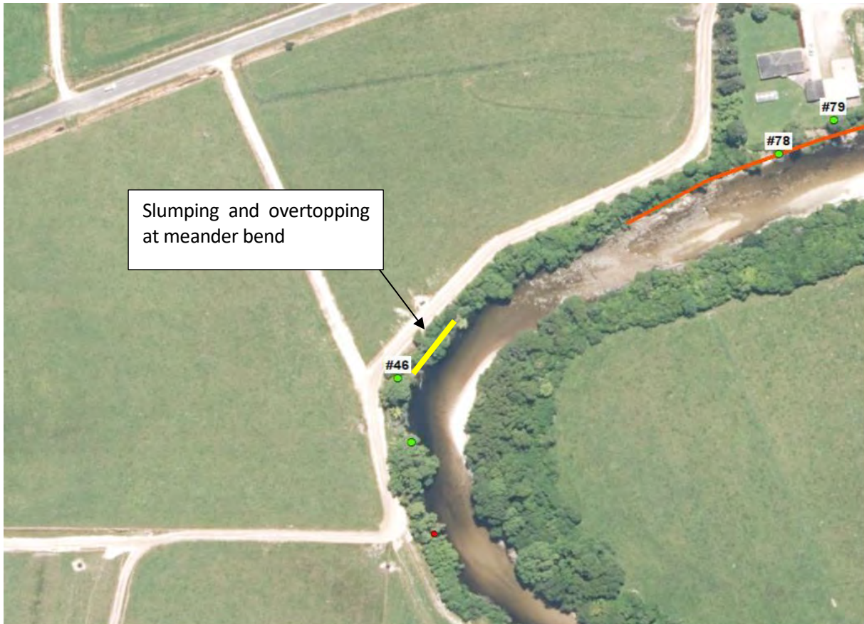
Photo 1: Location of erosion
