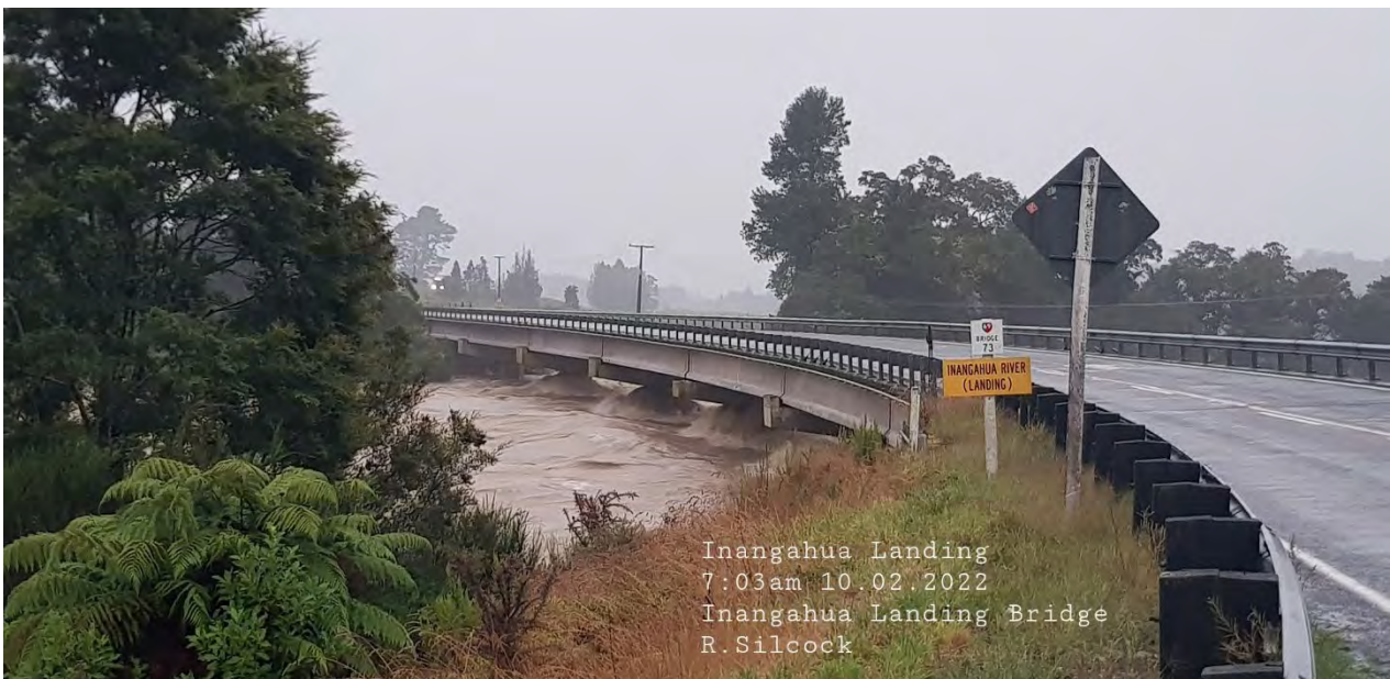
Photo 3 Inangahua River lapping the Bridge at Inangahua Landing
