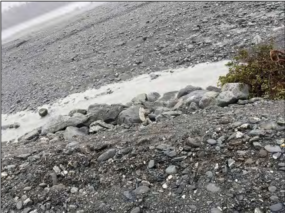
Rock work at toe of stop bank
