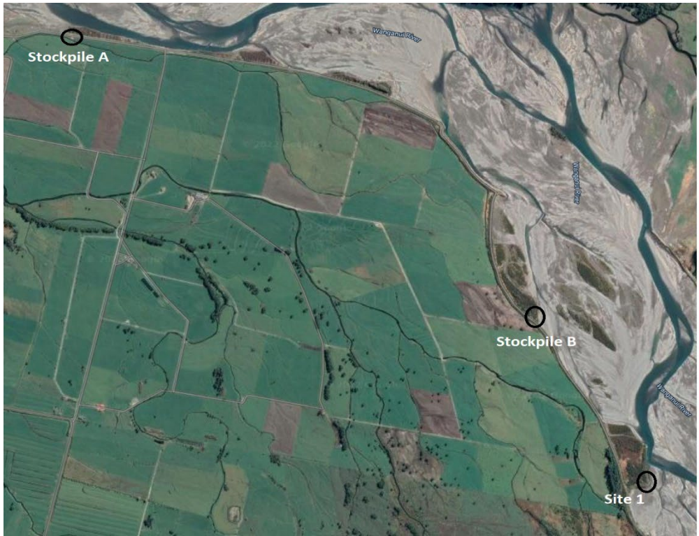
Locations of stockpiles A and B that will be replaced. Site 1 of minor riprap repairs needed to current Rating District Assets.
