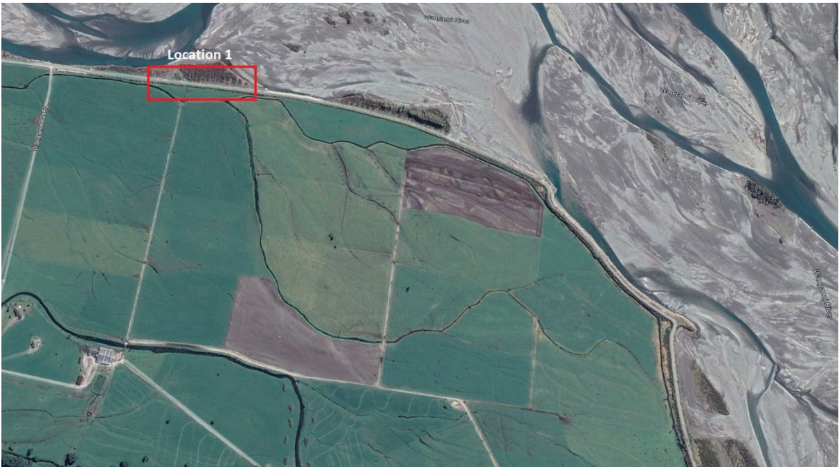
Location 1: Area where stopbank is being repaired and rock lined.
