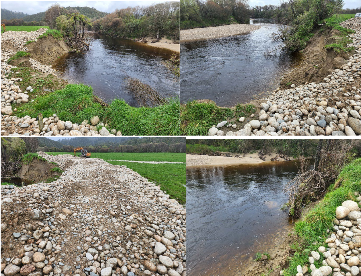
Temporary gravel bund in place for erosion protection at one site
