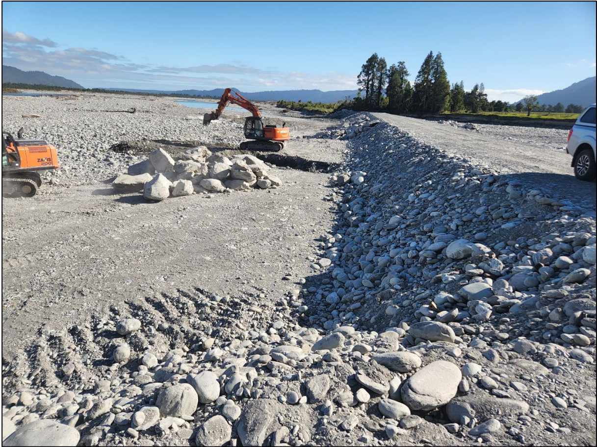
Looking downstream at newly constructed stopbank, groyne currently being constructed
