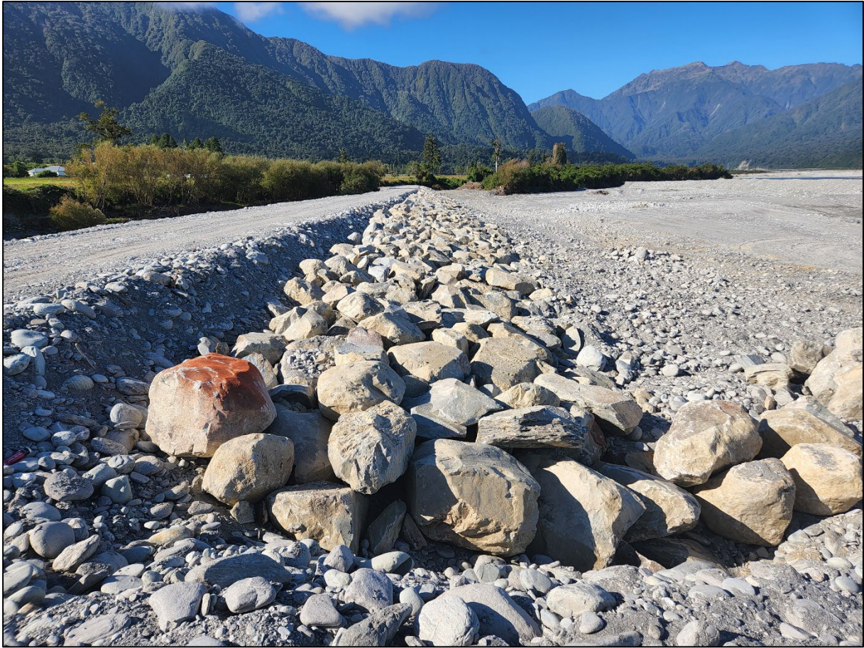
Looking upstream stream at newly constructed stopbank and rock riprap
