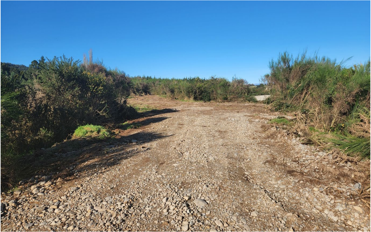
Photo 1. Cleared access to erosion scour
