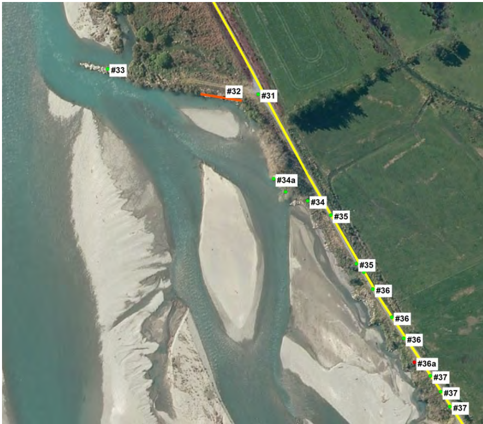
Site 4 – Damaged to Asset #33 requiring 280 tonnes of rock to remedy Site 5 – Damage to Asset #31 to 35 requiring 780 tonnes of rock to remedy Site 6 - Damage to Asset #35 to 37 requiring 780 tonnes of rock to remedy
